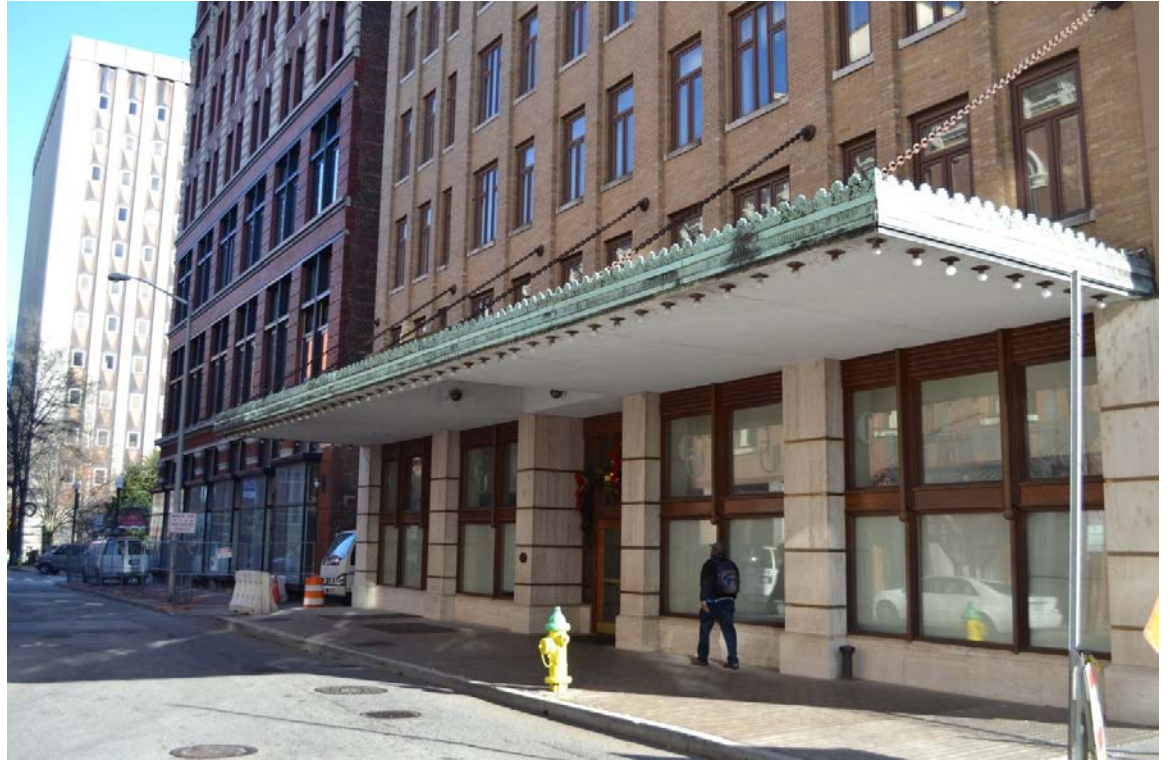
406 Union Ave awning
