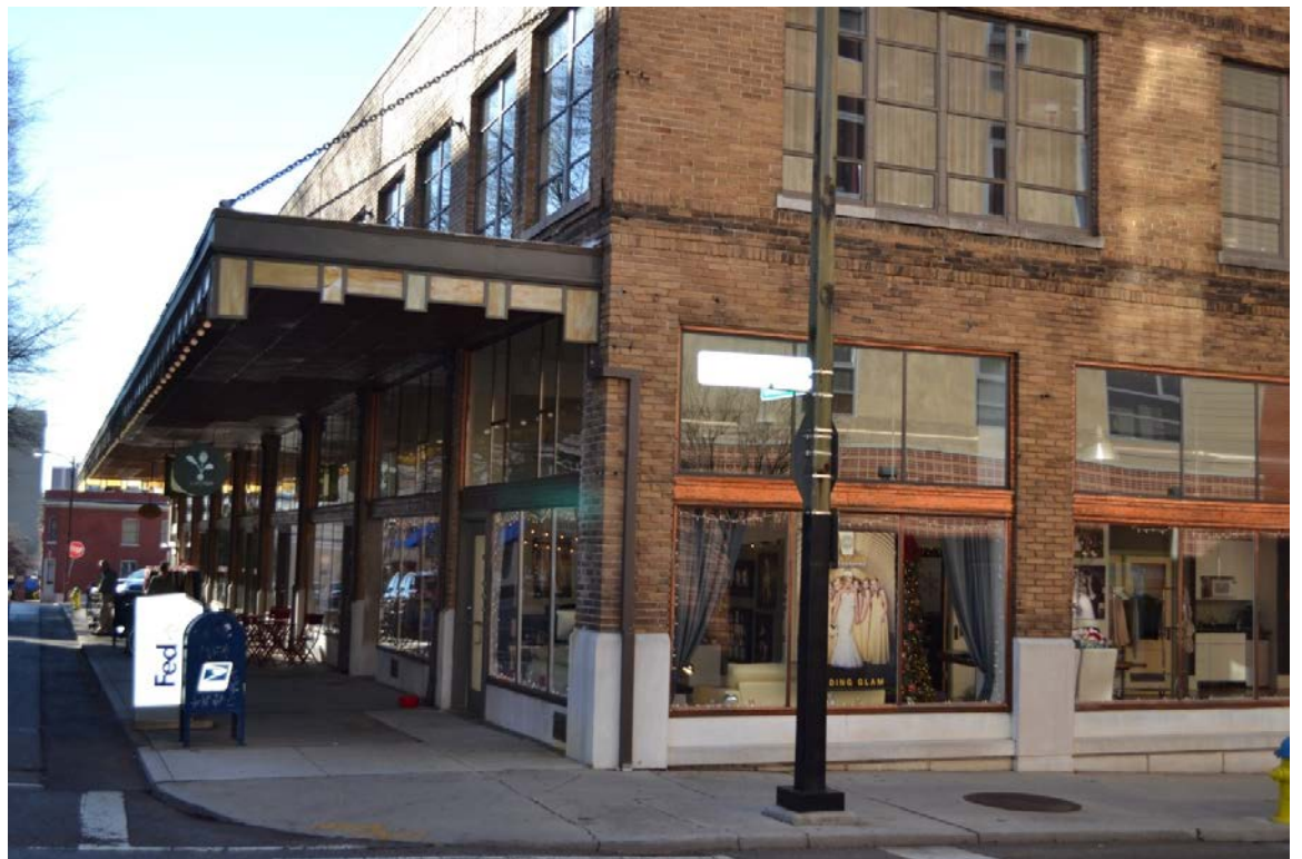
513 Union Ave awning
