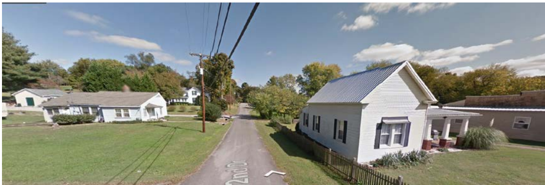
Views of previous house on the 10817 2 nd Drive site (in background), now demolished.
