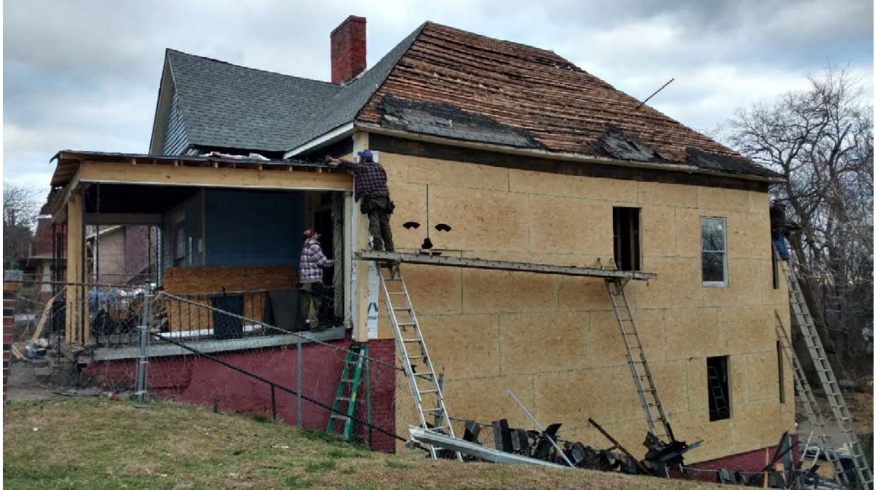
412 E. Scott - Re-sheathing in progress on south side
