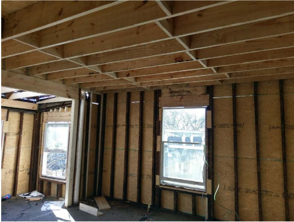
412 E. Scott - Windows on 2nd-level south from interior showing new headers
