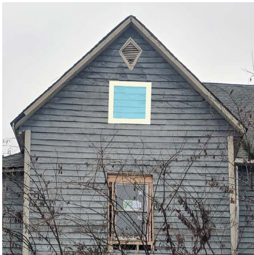
412 E. Scott north gable simulation as proposed. Relocate vent higher in gable and add square 30x30 square window for egress.
