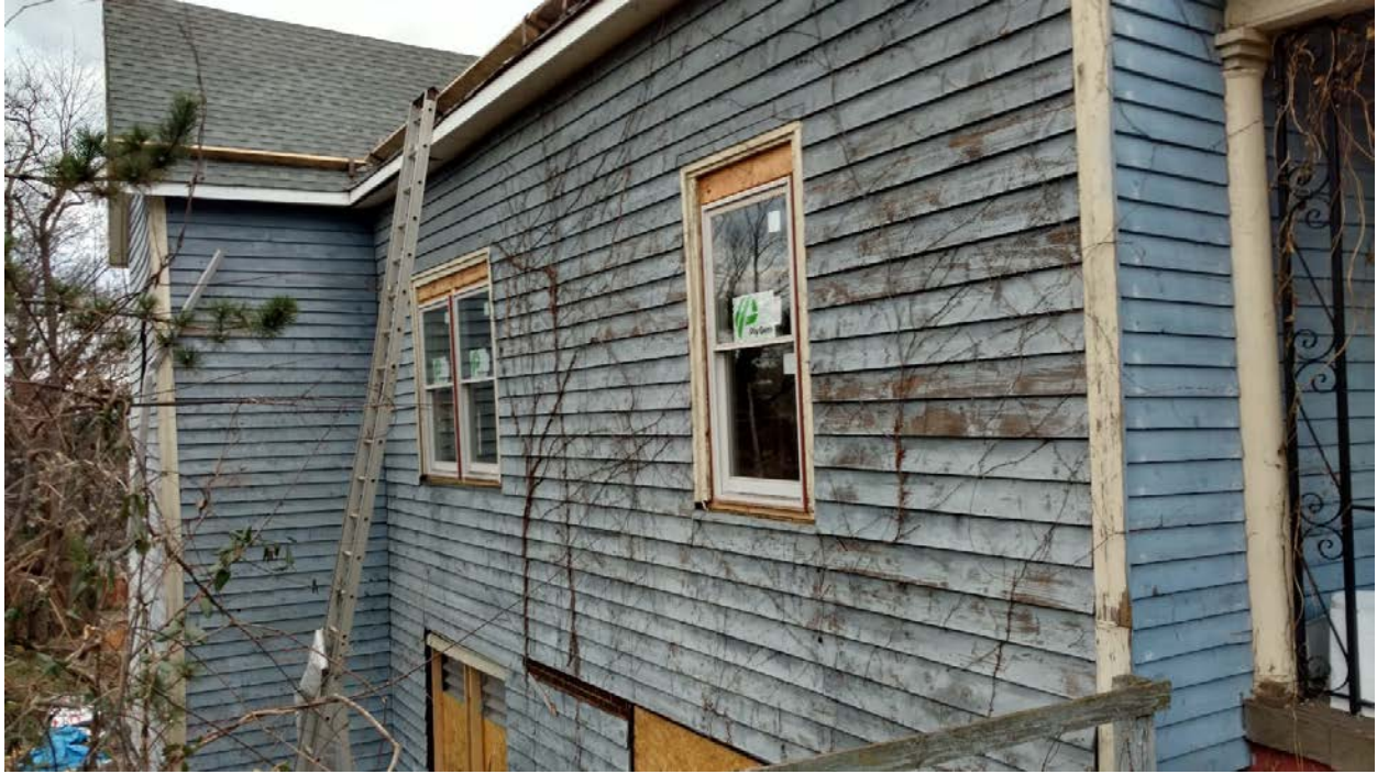
412 E. Scott - Replacement windows on north side showing infill
