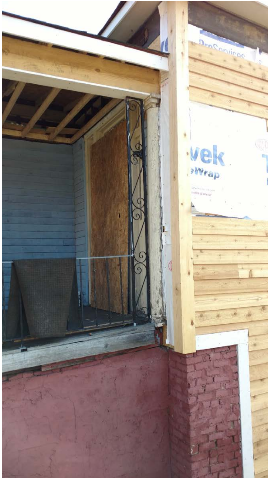
412 E. Scott - SW (Front) corner of house showing south siding does not meet up with siding on front
