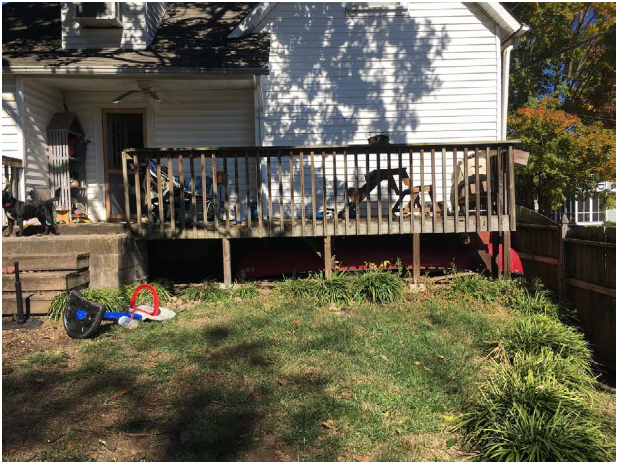
View of Existing Deck from Rear
