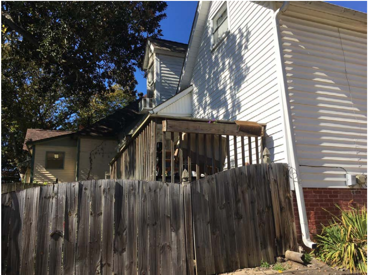
View of Existing Deck from East Side of the House
