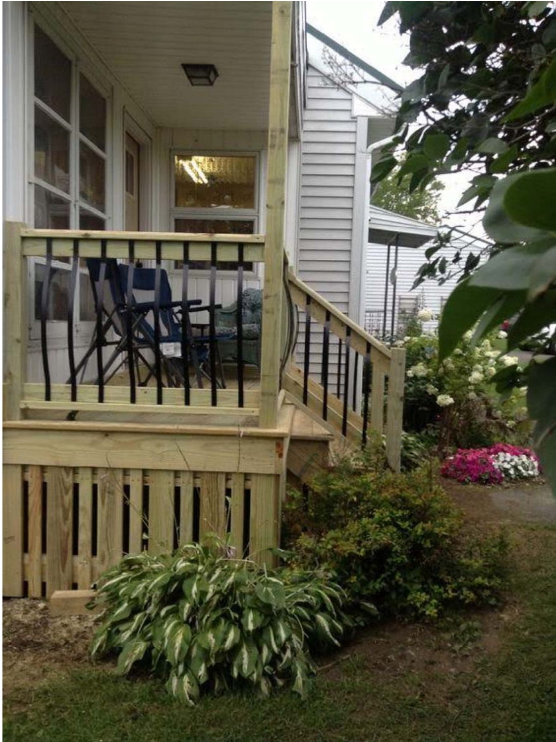
610 Caswell - Vertical underpinning
