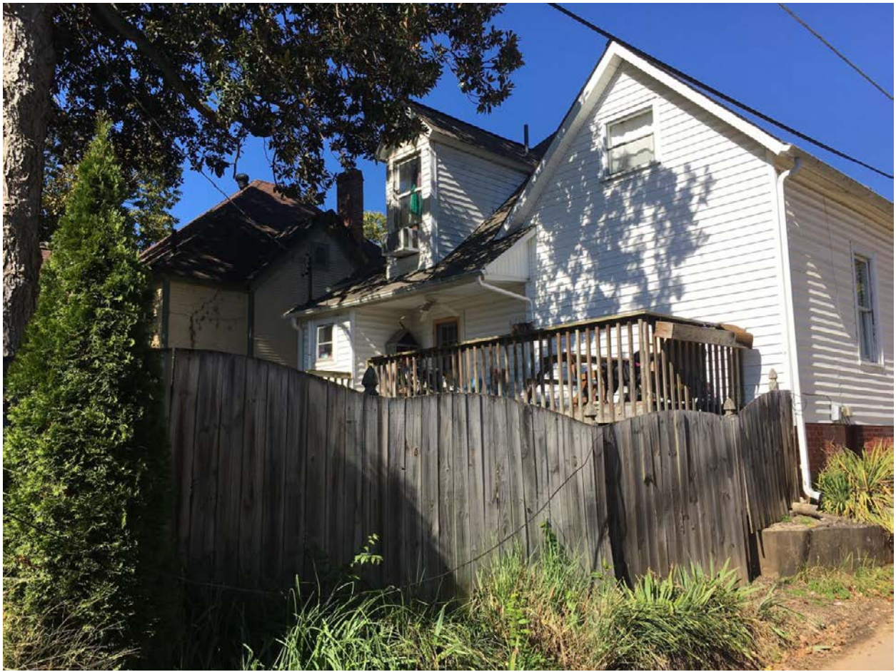
View of Existing Deck from Alley
