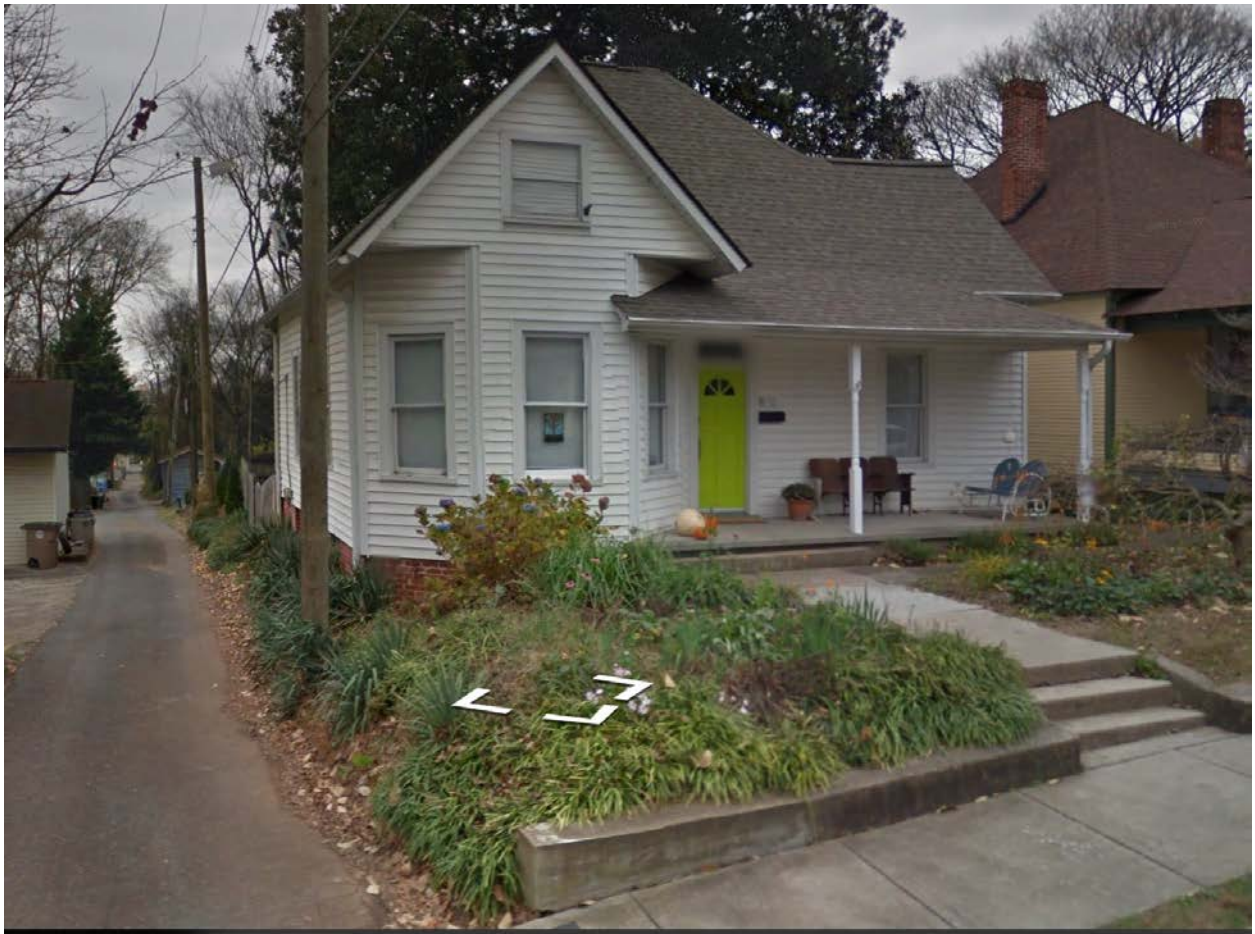
610 Caswell Street Front Façade and Alley to the East
