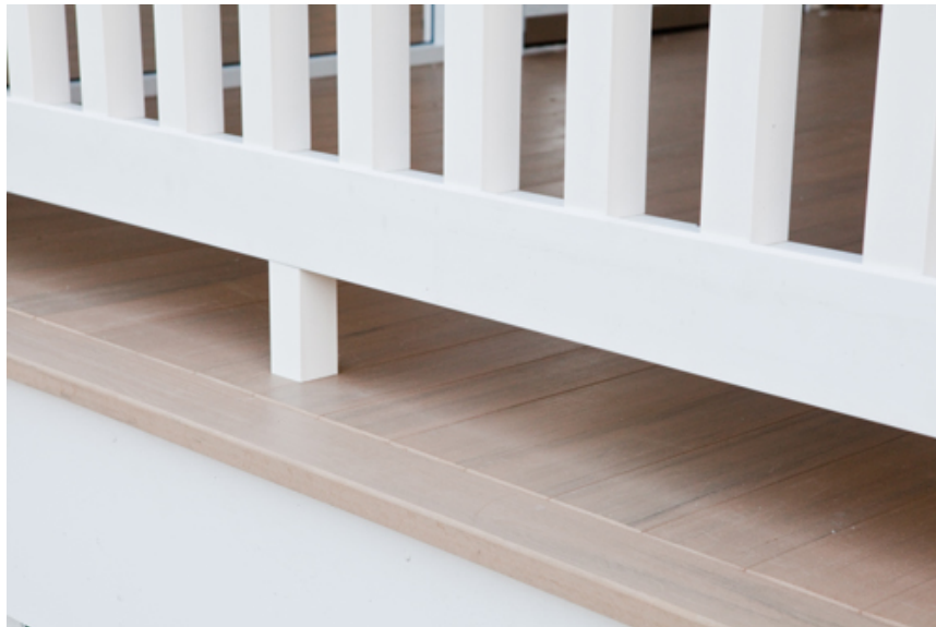
Aeratis PVC tongue-and-groove composite flooring showing 1x4 trim on edge
