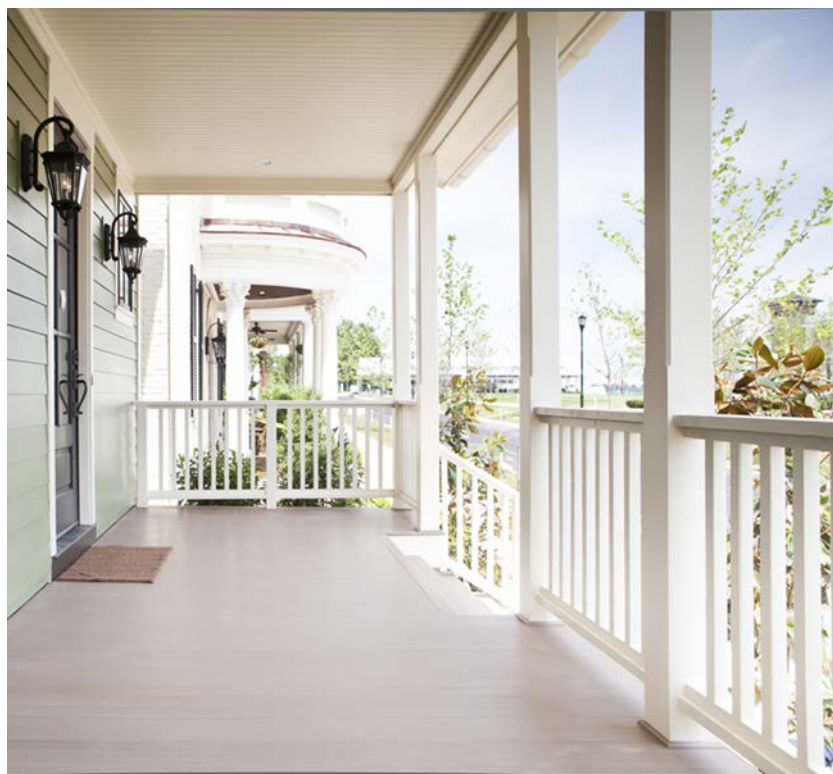
Aeratis PVC porch balustrade installation
