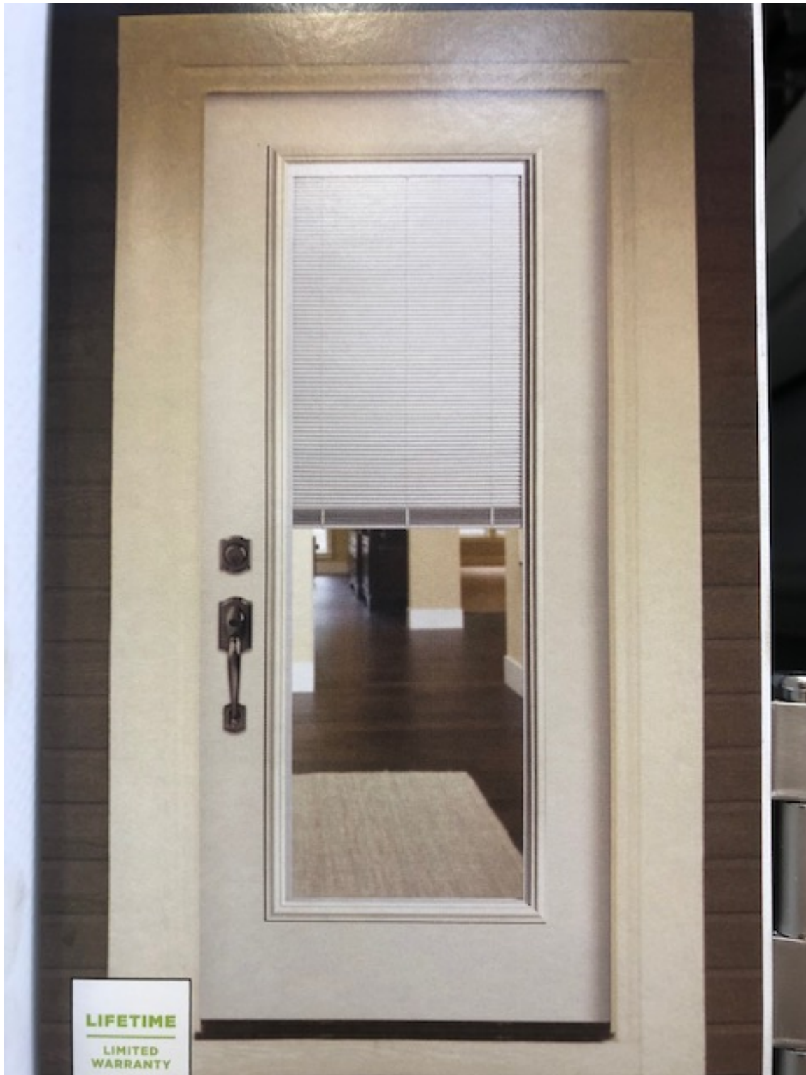
1413 Highland – Second floor door
