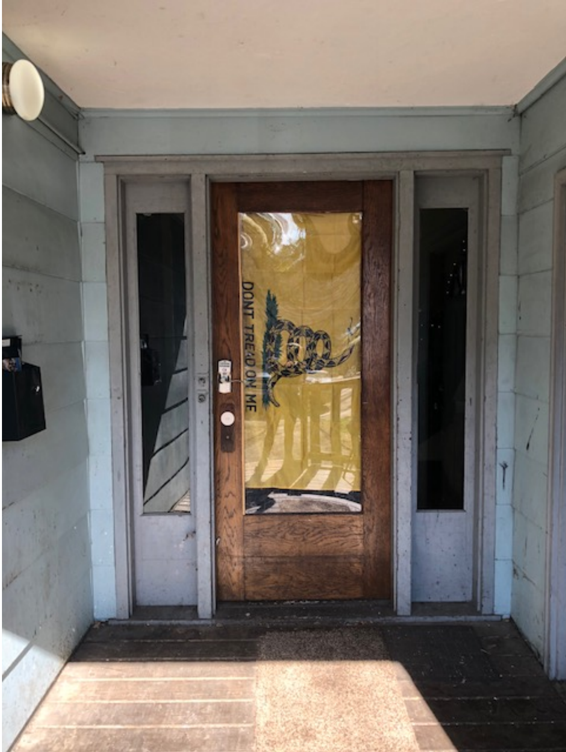
1413 Highland – Front door
