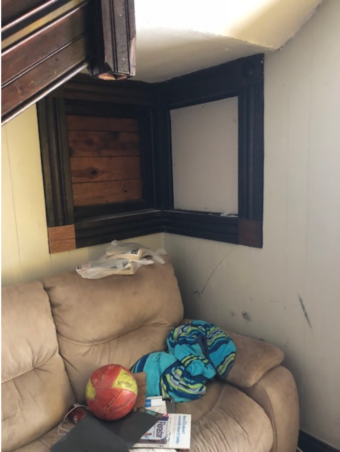
1413 Highland - Corner windows from the interior
