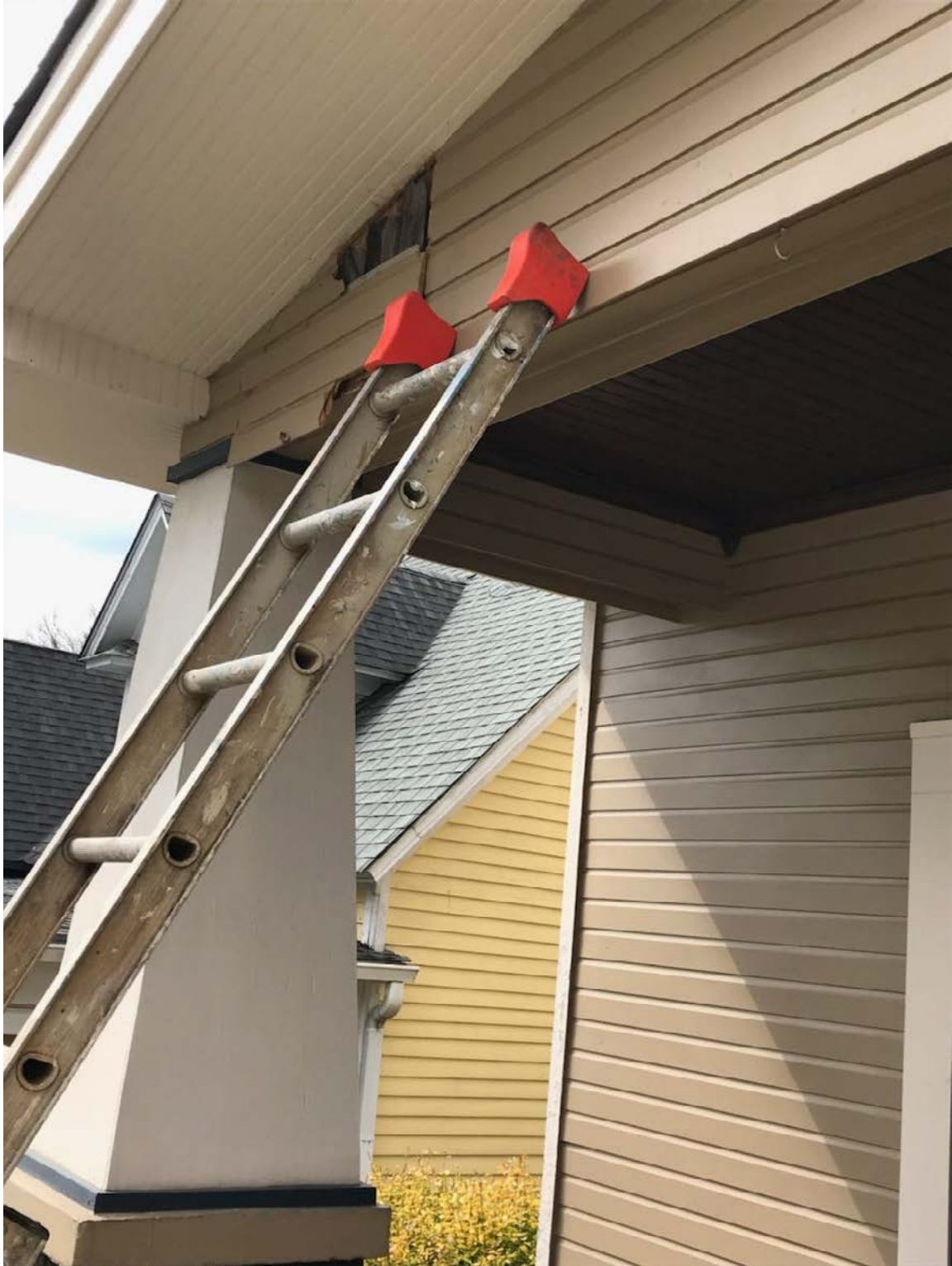
809 Eleanor - Removed siding in front porch gable showing shingles
