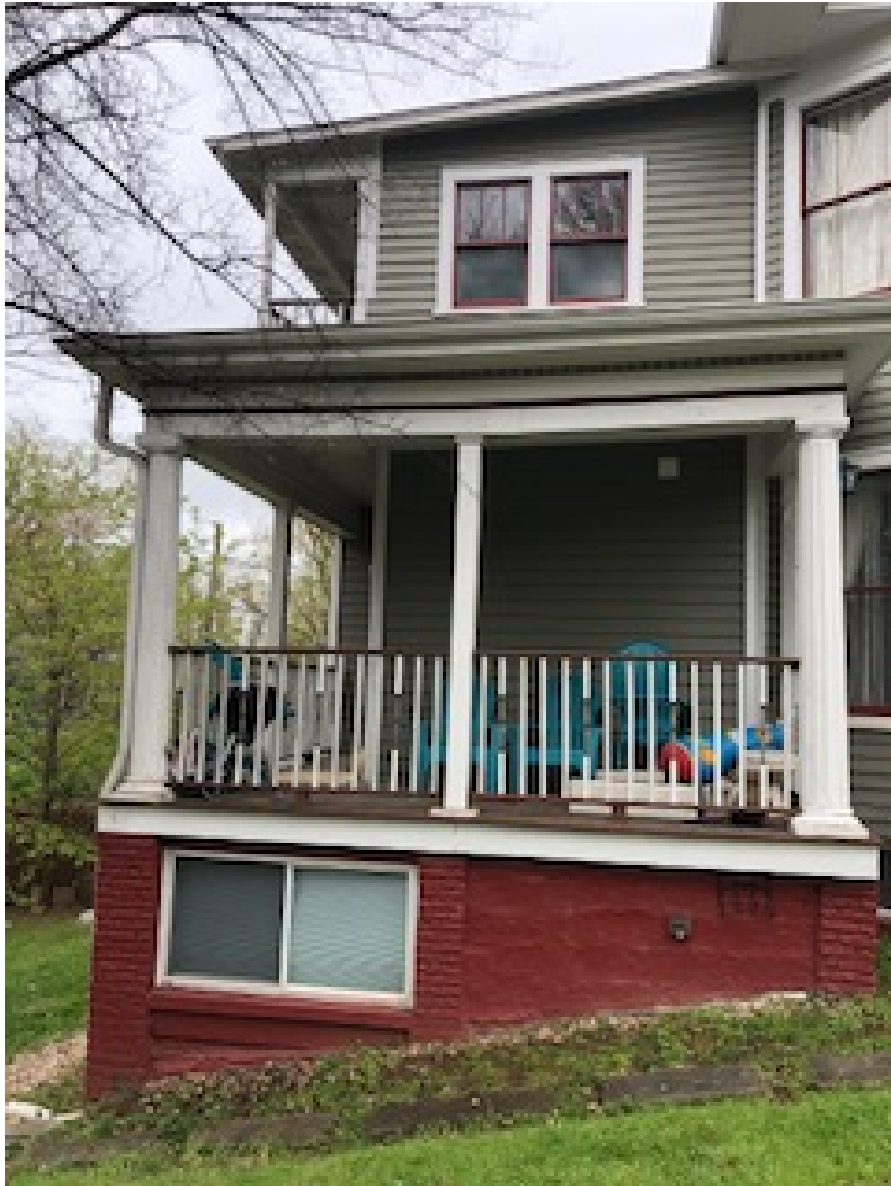
940 Eleanor - North side of wrap-around back porch
