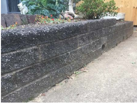
Existing retaining wall
