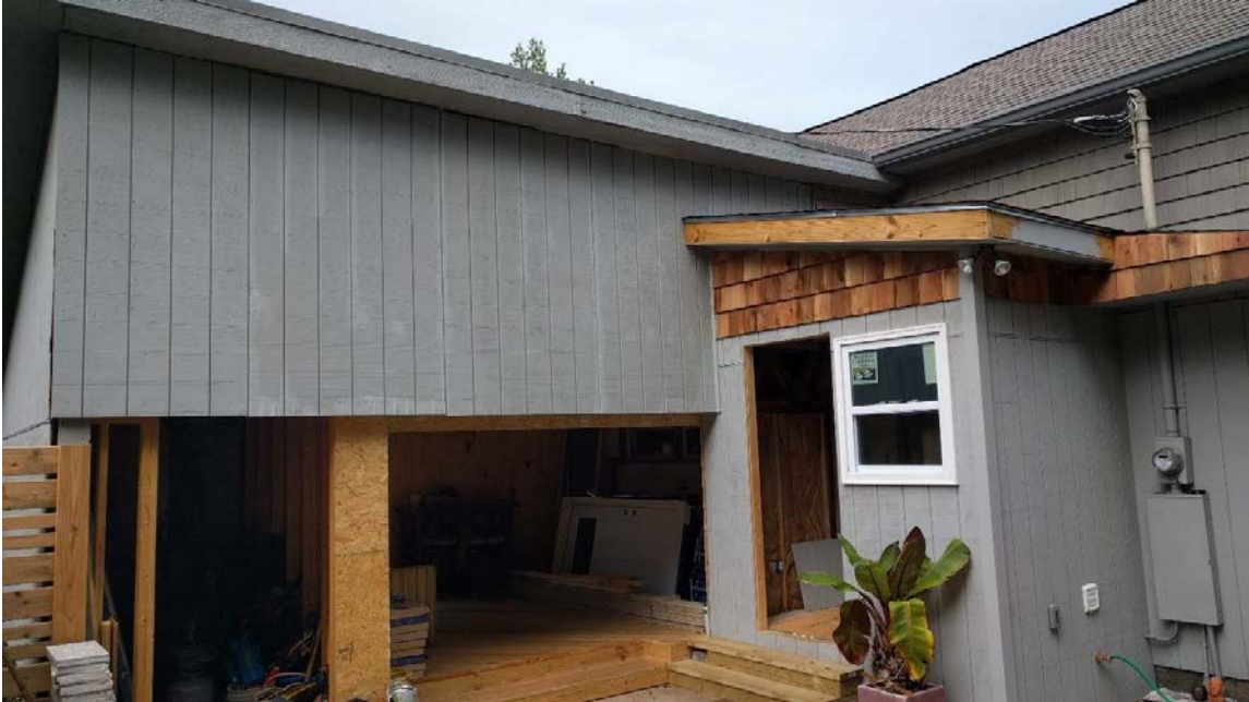
Overall view of the back
