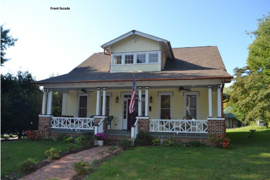
1012 Oak Ave - Front façade
