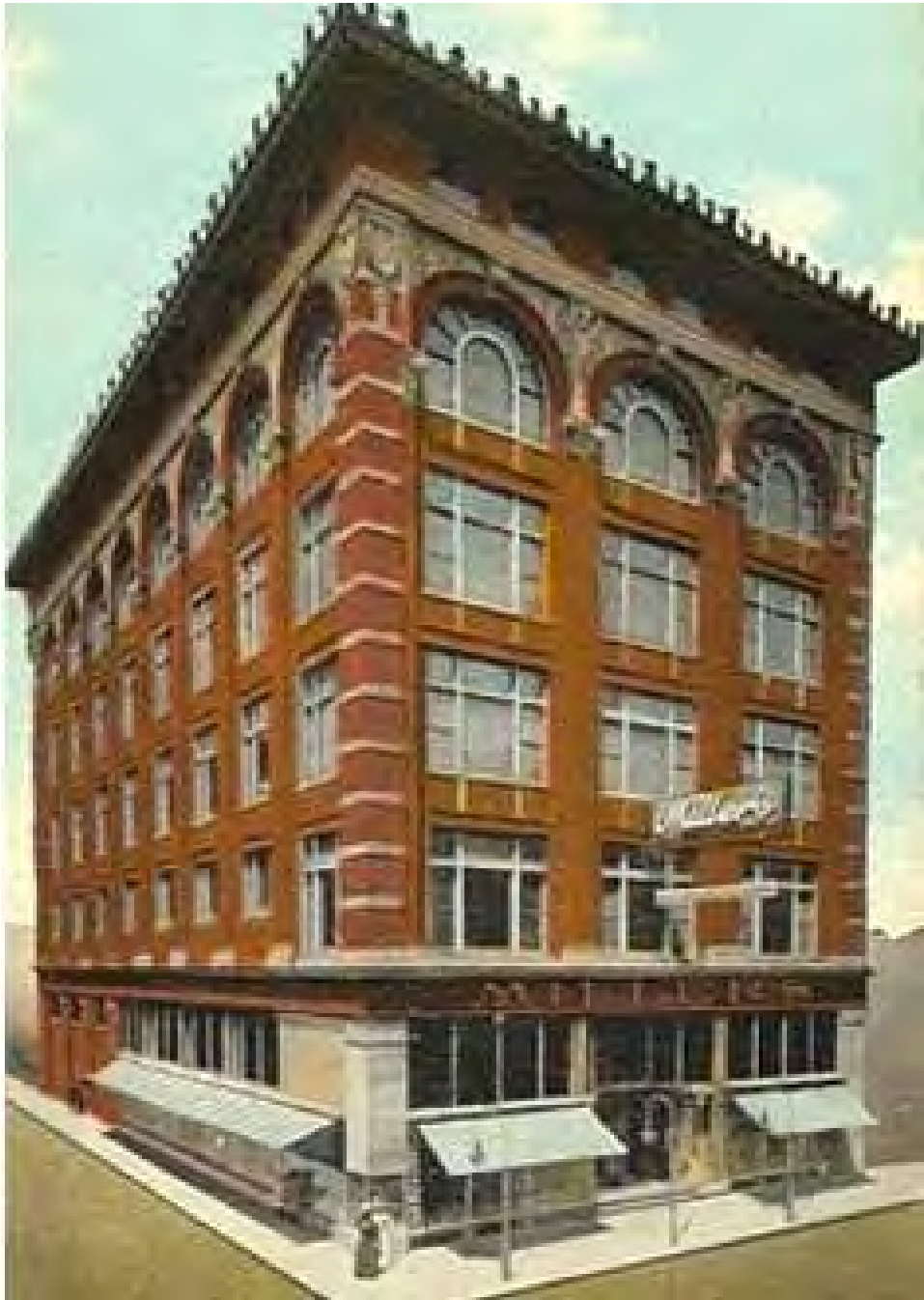
Miller Building showing projecting sign
