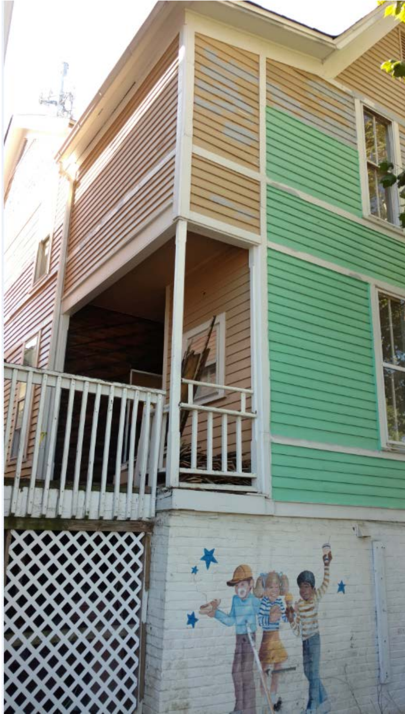
Rear of 404 11 th showing cut-away porch
