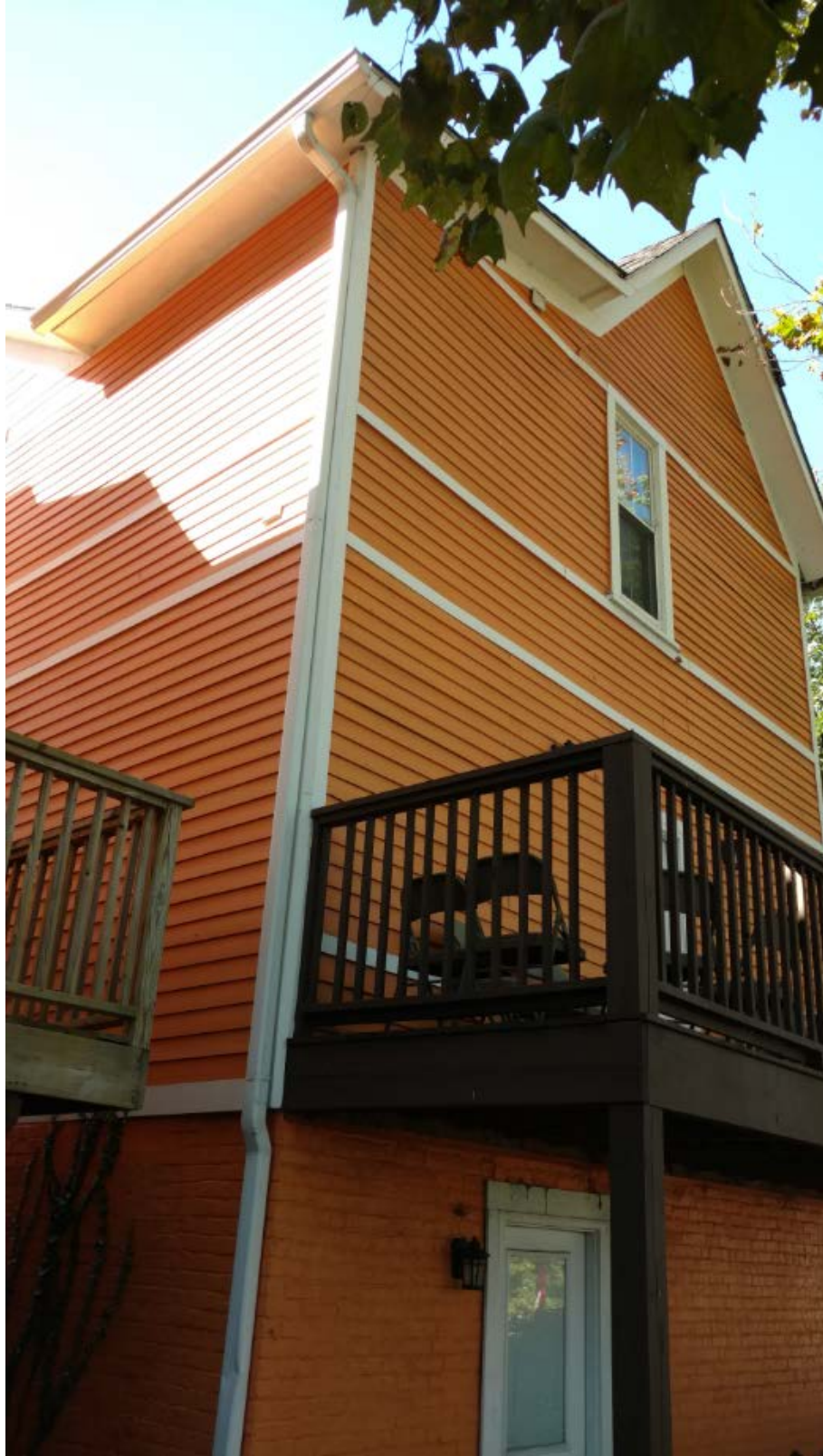
Rear of 402 11 th showing enclosure of cut-away porch
