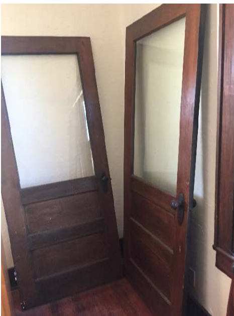
Original set of doors proposed to be re-installed in center of rear porch
