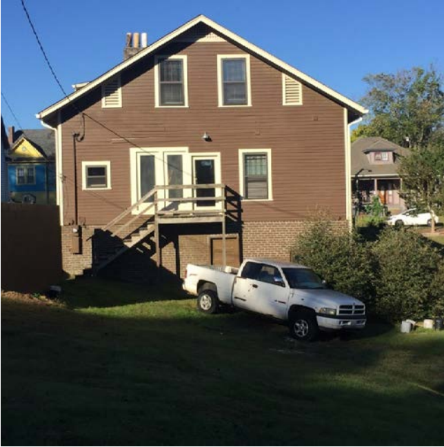
1012 Gratz Street current rear façade showing inappropriate set of doors
