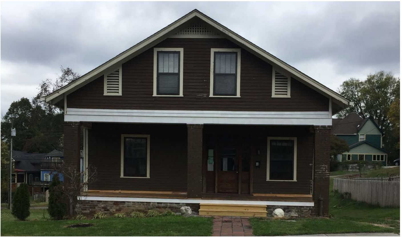
1012 Gratz Street current front facade
