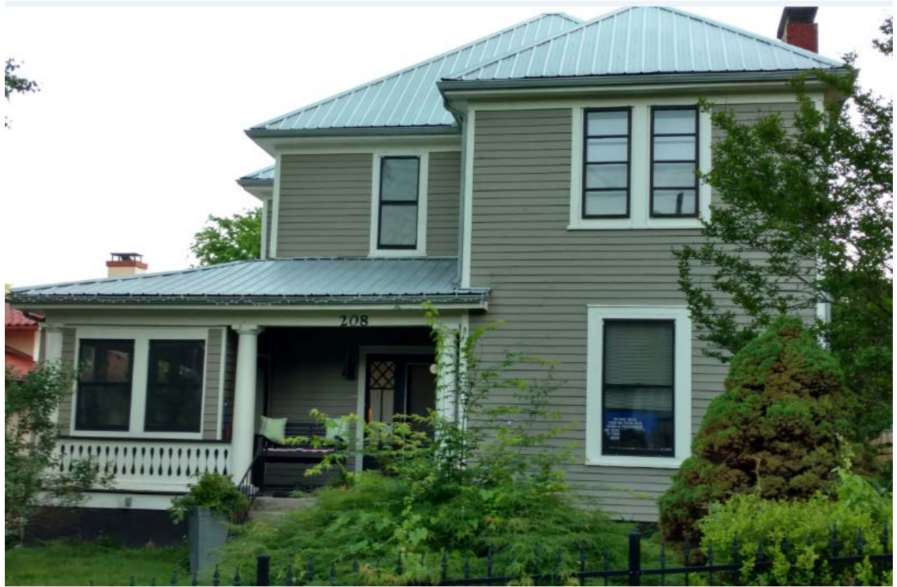
208 W. Glenwood Avenue – ribbed metal roofing approved 2009
