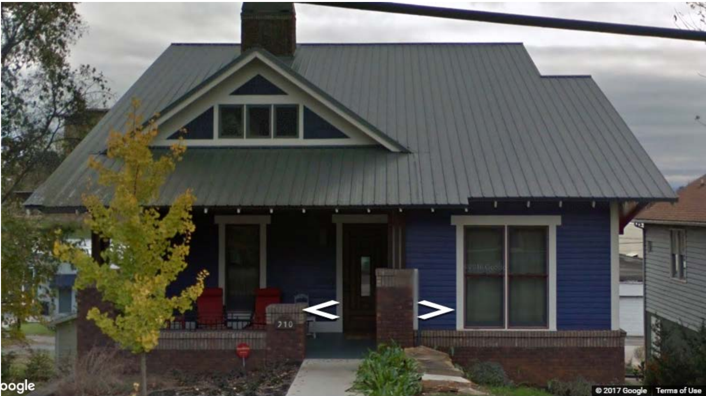
310 E. Oklahoma Avenue in ONK with ribbed metal roofing – late construction (HZC approved)
