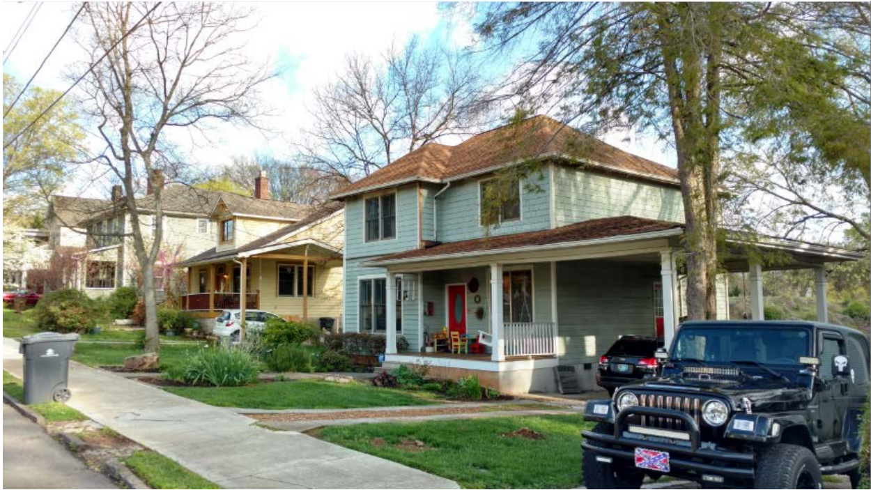
1335 Grainger Avenue looking northwest in the streetscape
