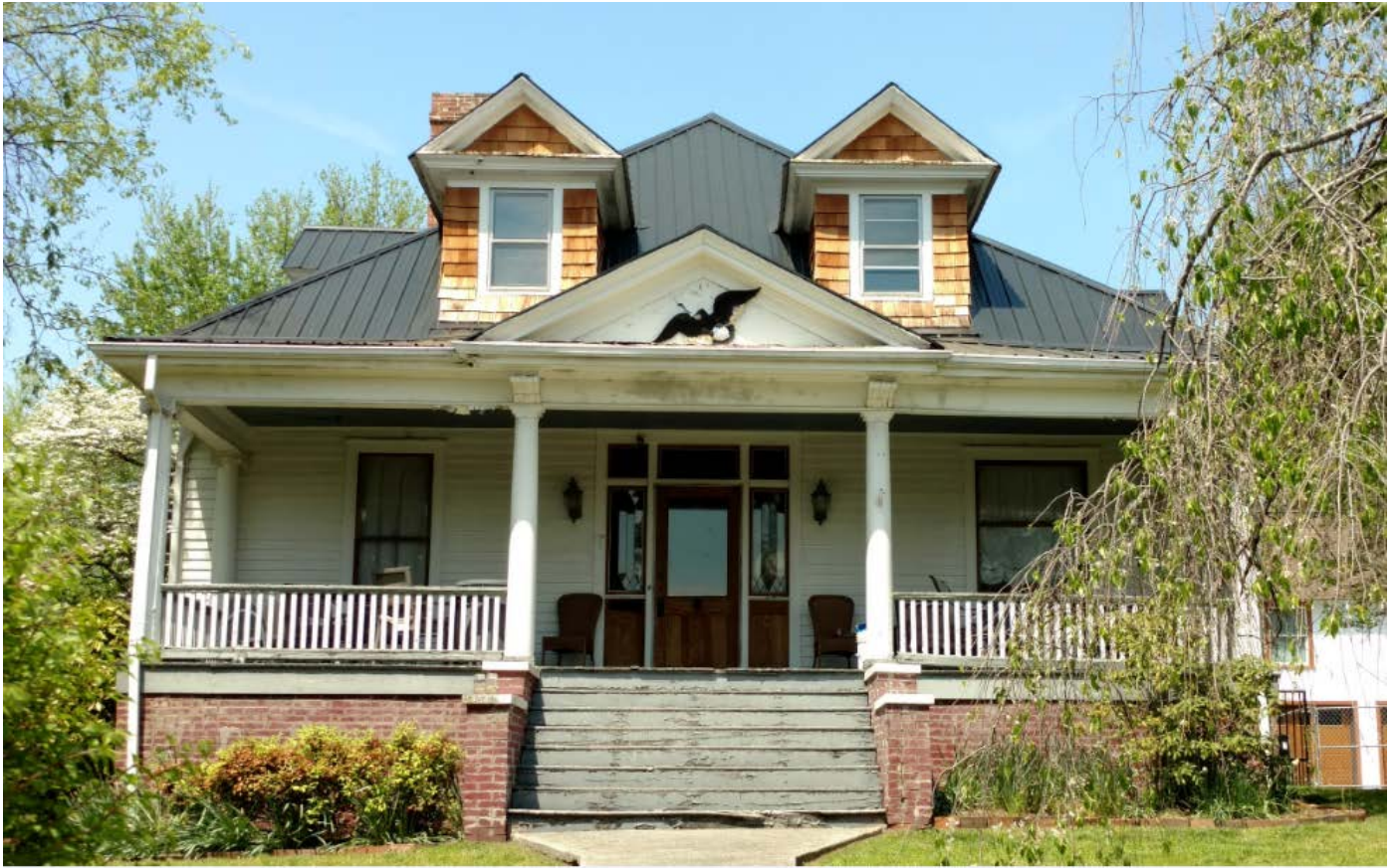
410 E. Scott Avenue in ONK with ribbed metal roofing (no COA)
