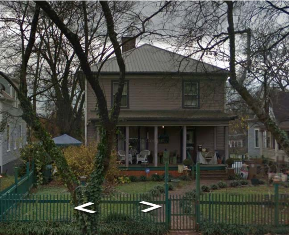
244 E. Oklahoma Avenue in ONK with ribbed metal roofing (HZC approved)
