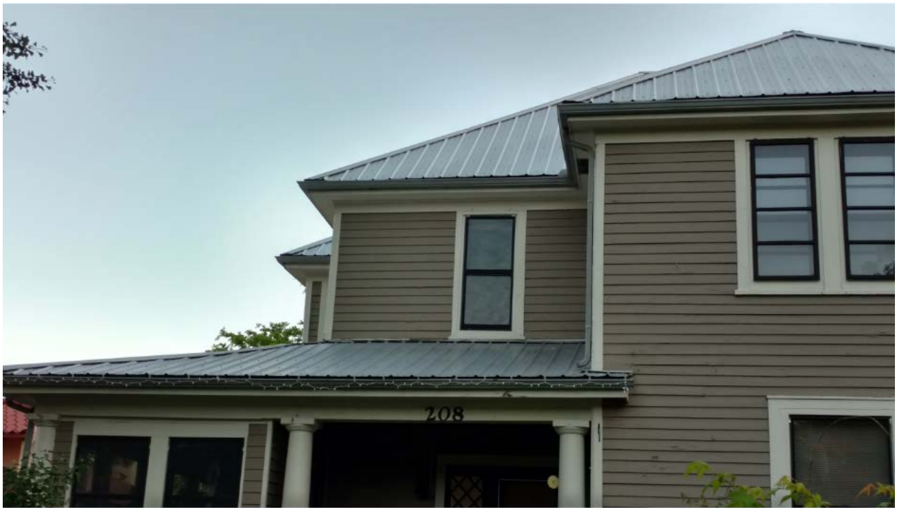
208 W. Glenwood Ave close-up approved by HZC 2009
