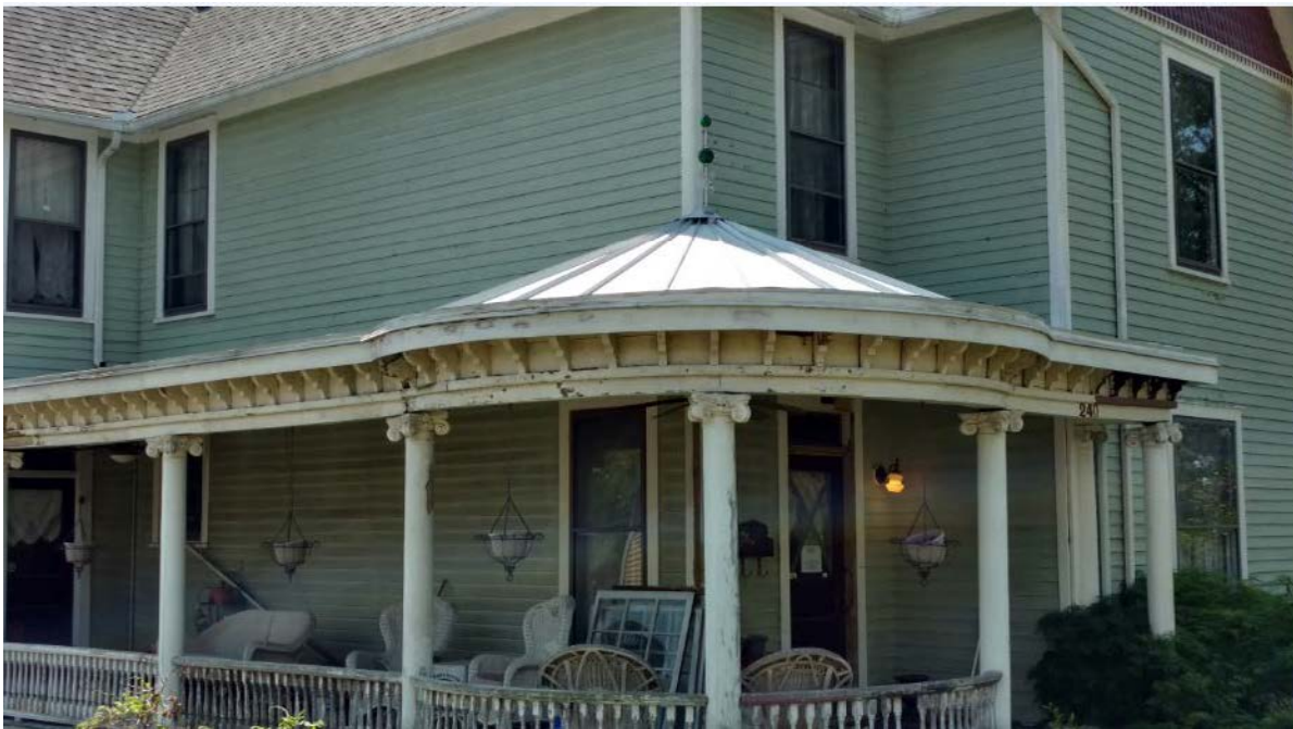
240 E. Scott Avenue in ONK with standing seam metal roof on porch only (HZC approved)
