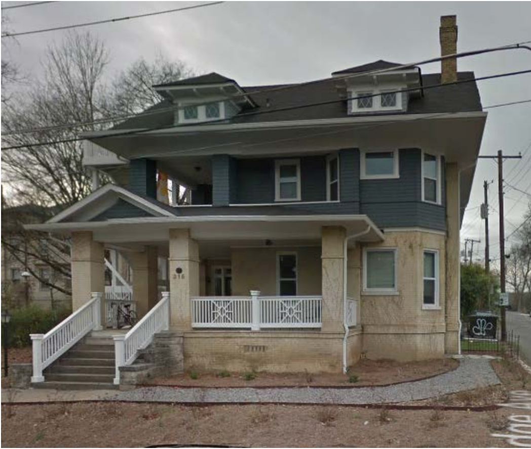
315 James Agee Street rear and NW façade
