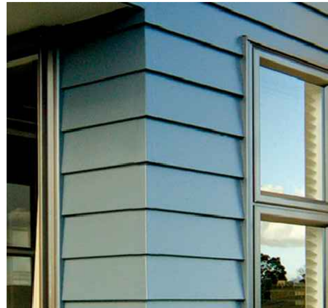
4 Proposed Artisan Siding w/ Mitered Corners SCALE: 1/8" = 1'-0"
