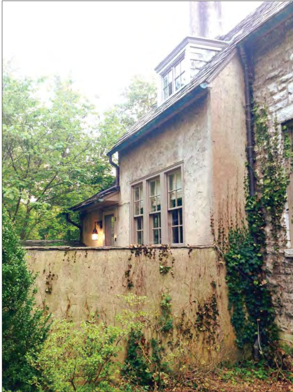
4 - Left Side View / Rear Entry
