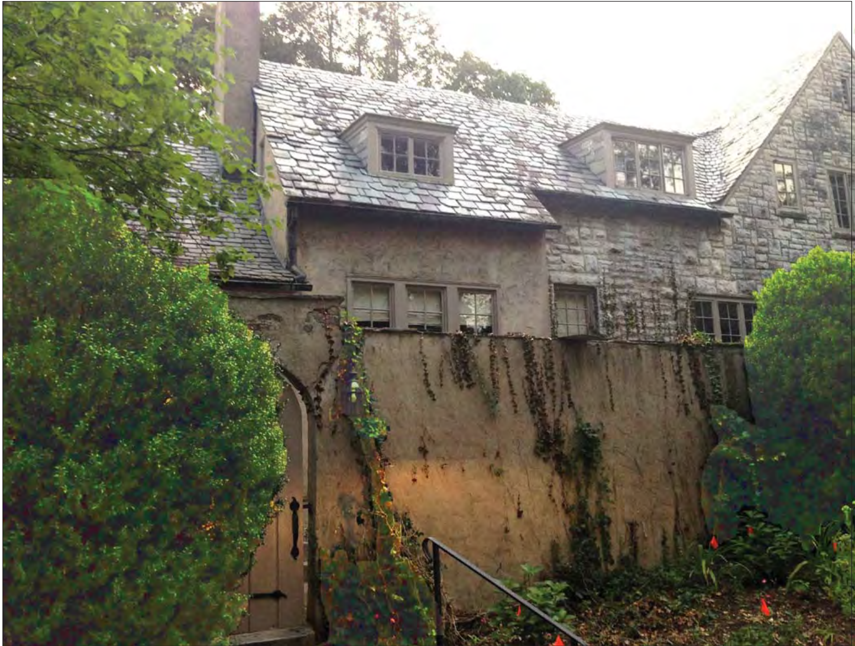
3 - Left Side View / Rear Entry
