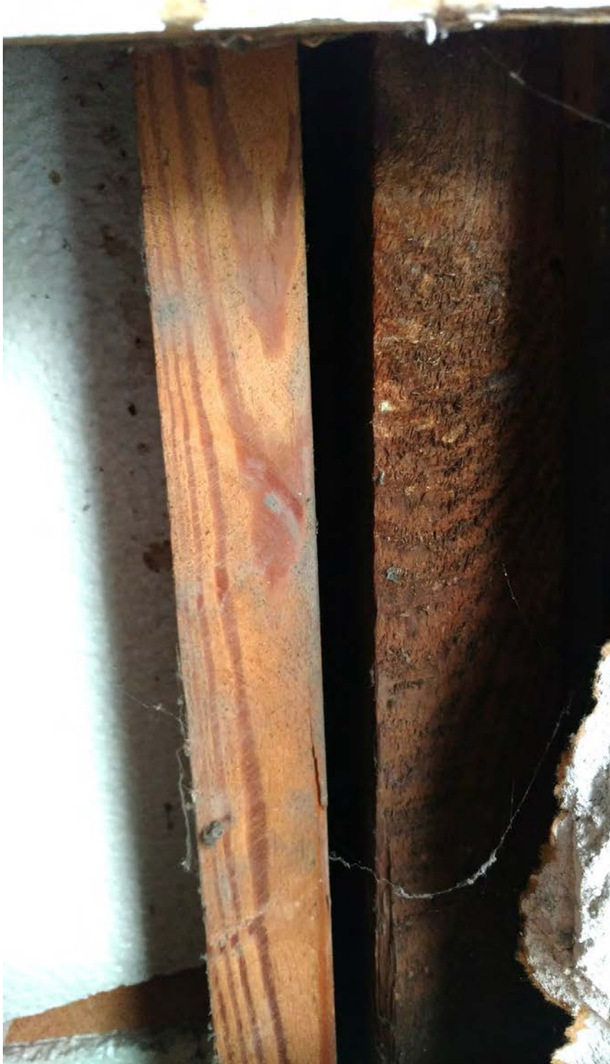
1424 Freemont – Old and new studs at front door
