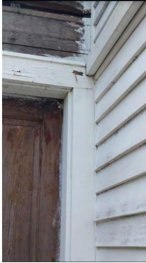
1424 Fremont – Non-original door on north side, facing toward the front. Indication of door inserted into previously existing sided wall projection
