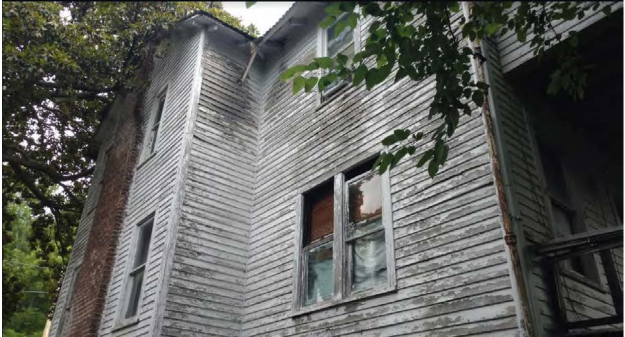
1424 Fremont – Overall south façade looking toward the front
