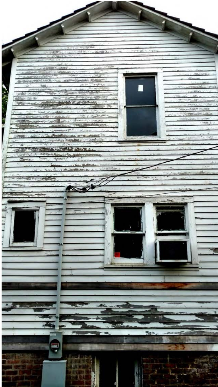
1424 Fremont – North façade showing small fixed window to be removed.
