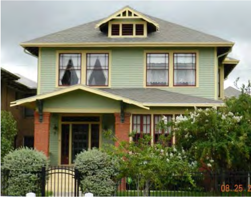
Four-square with off-center front-gabled stoop similar to subject house with transom & sidelights
