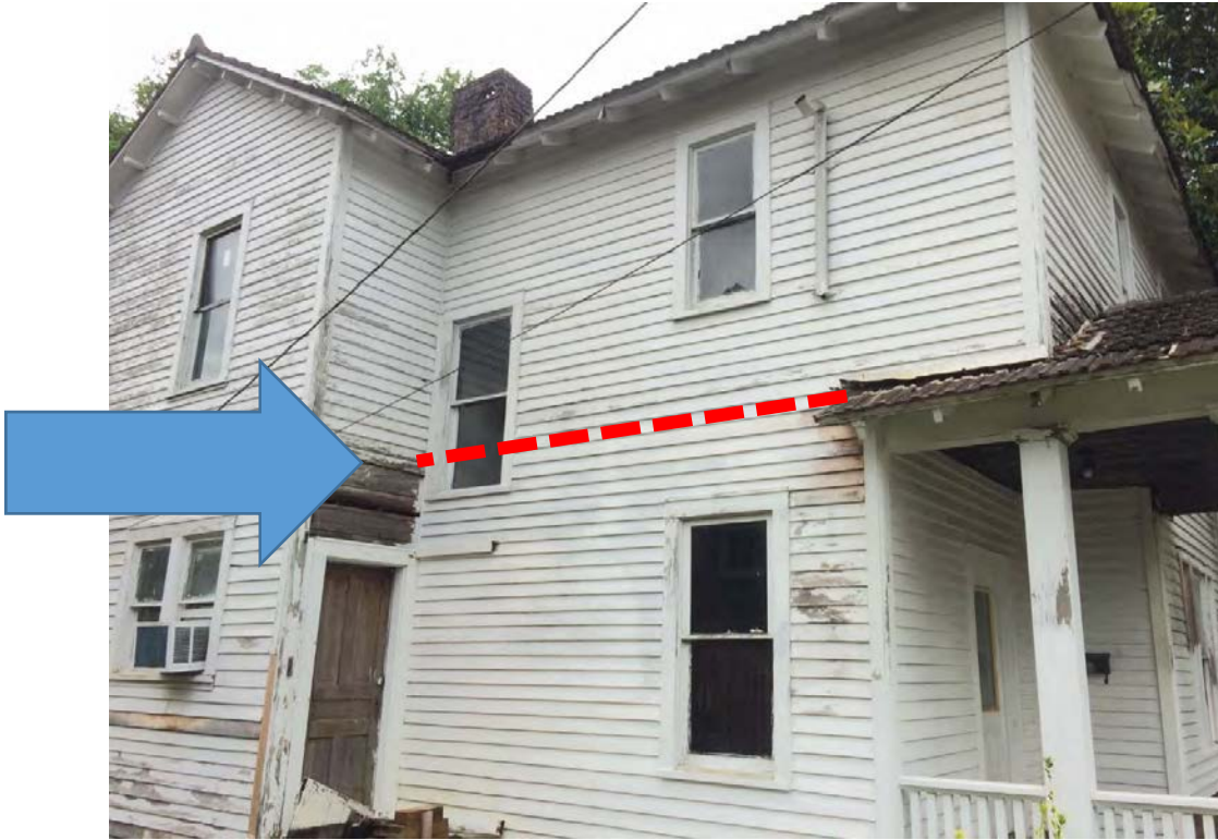
A wrap around porch (which would support a side door) would have traversed the lower staircase window.
