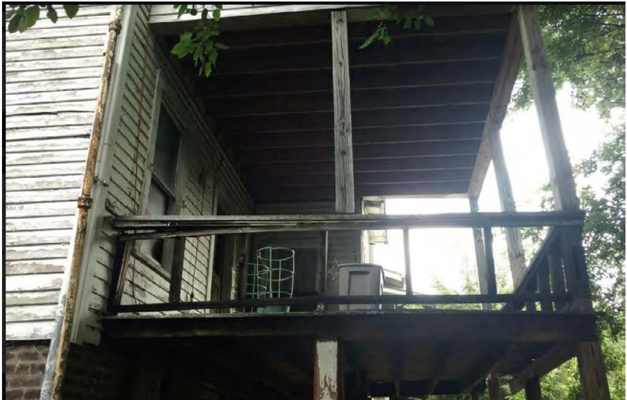
View of rear decks from south side
