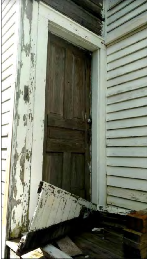
1424 Fremont – Non-original door on north side, facing toward the front. Indication of door inserted into previously existing sided wall projection
