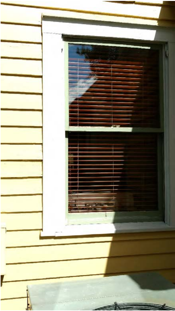
Close-up view of window to be removed
