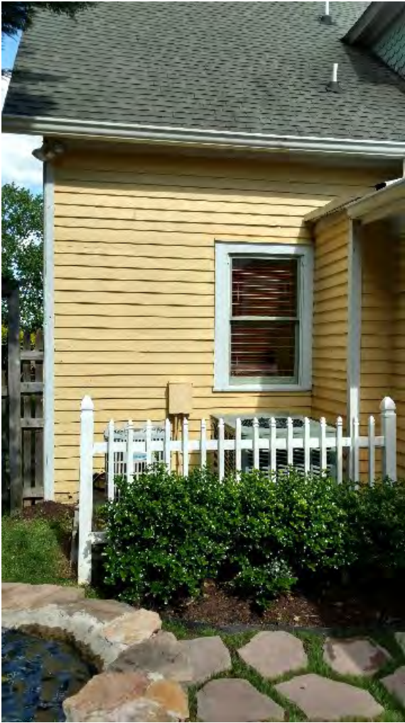
View of overall wall where doors are proposed to be installed
