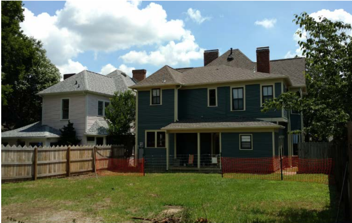
1019 Eleanor Street rear elevation showing location of garage to the right along alley
