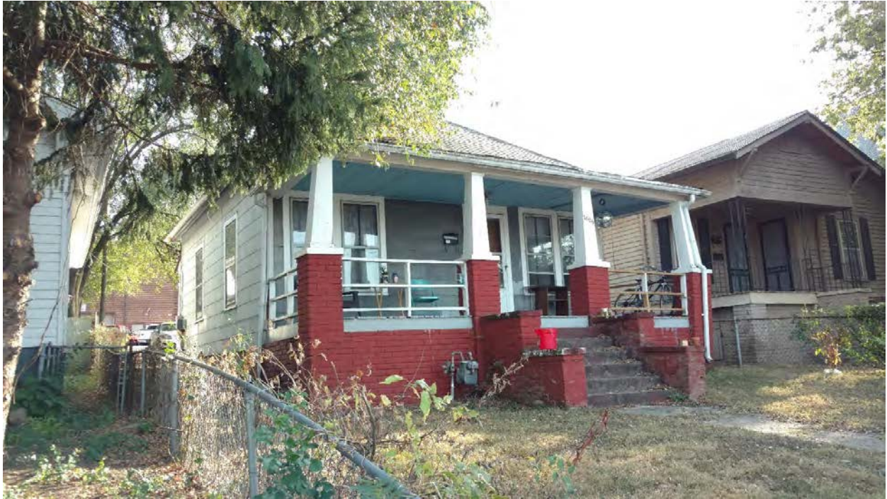
1626 Forest Ave - Front facade looking southwest
