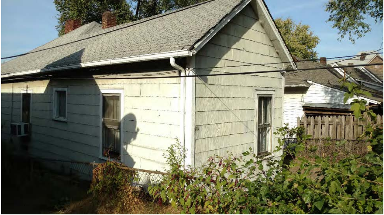
1626 Forest Ave - West facade looking northeast
