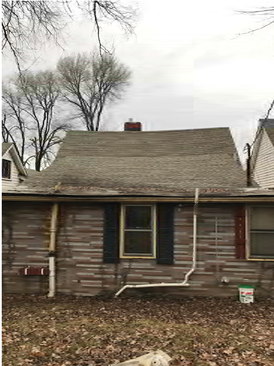
1618 Forest Ave - Rear view - looking North
