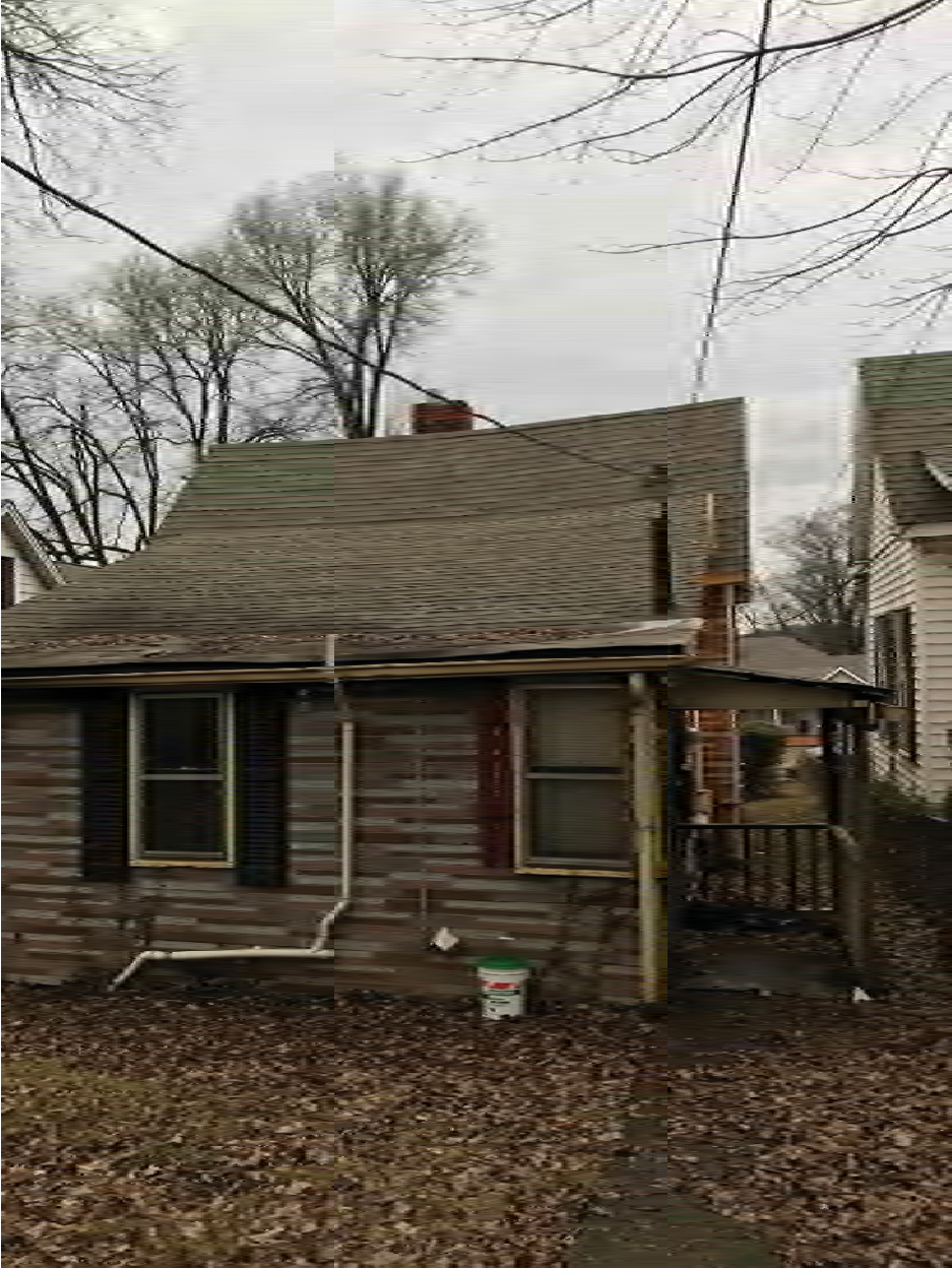
1618 Forest Ave - Rear view - looking North
