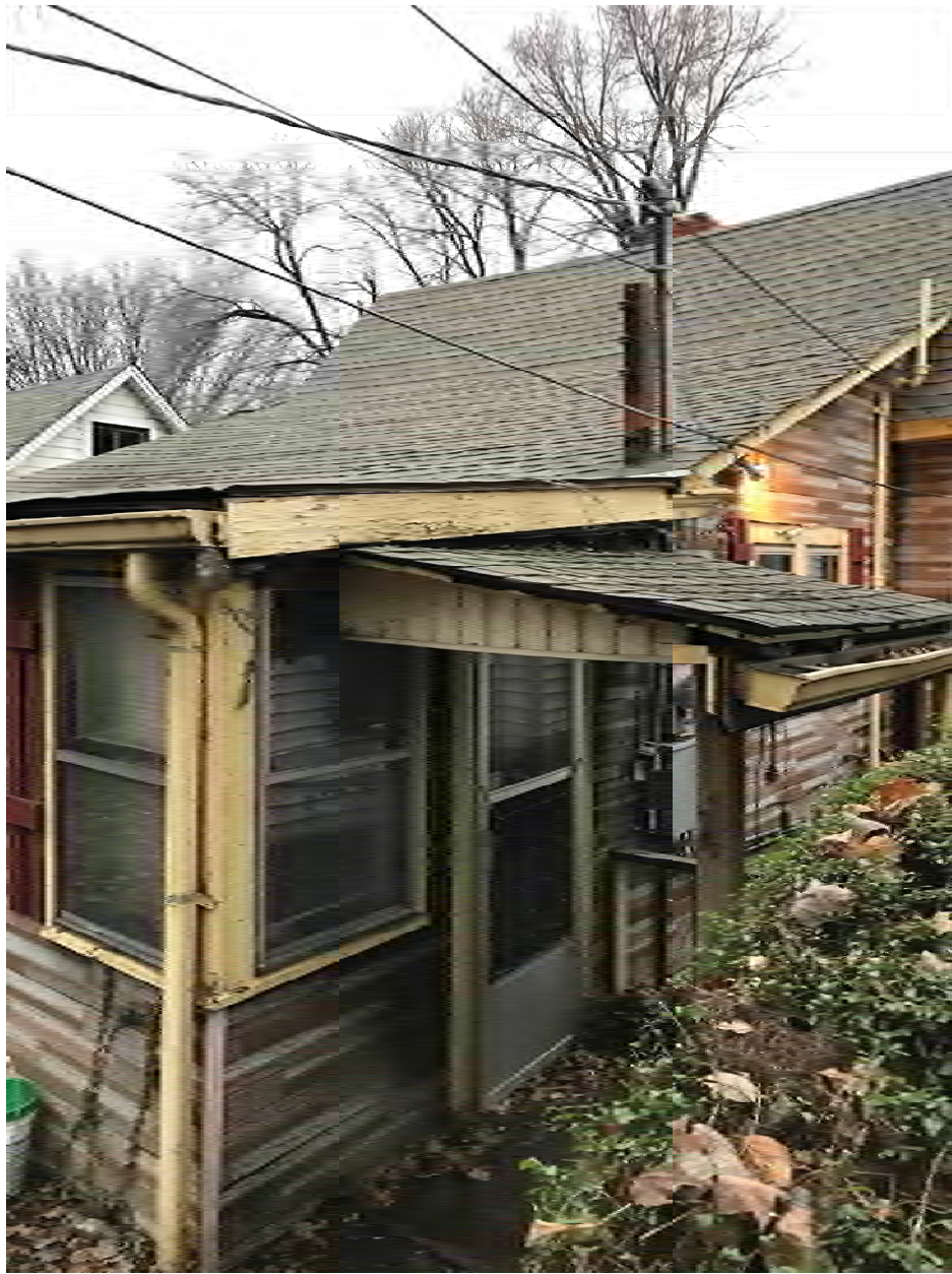
1618 Forest Ave - Rear side view - looking West
