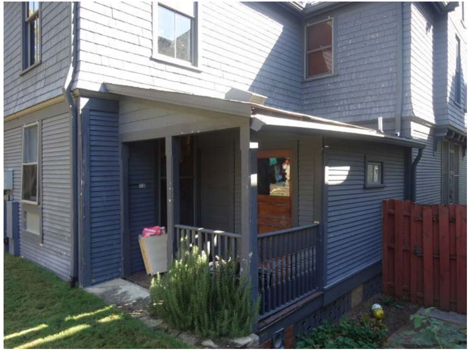
Existing mudroom on south side
