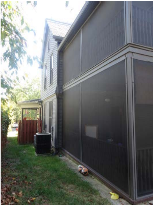
Two-story screen porch on north side
