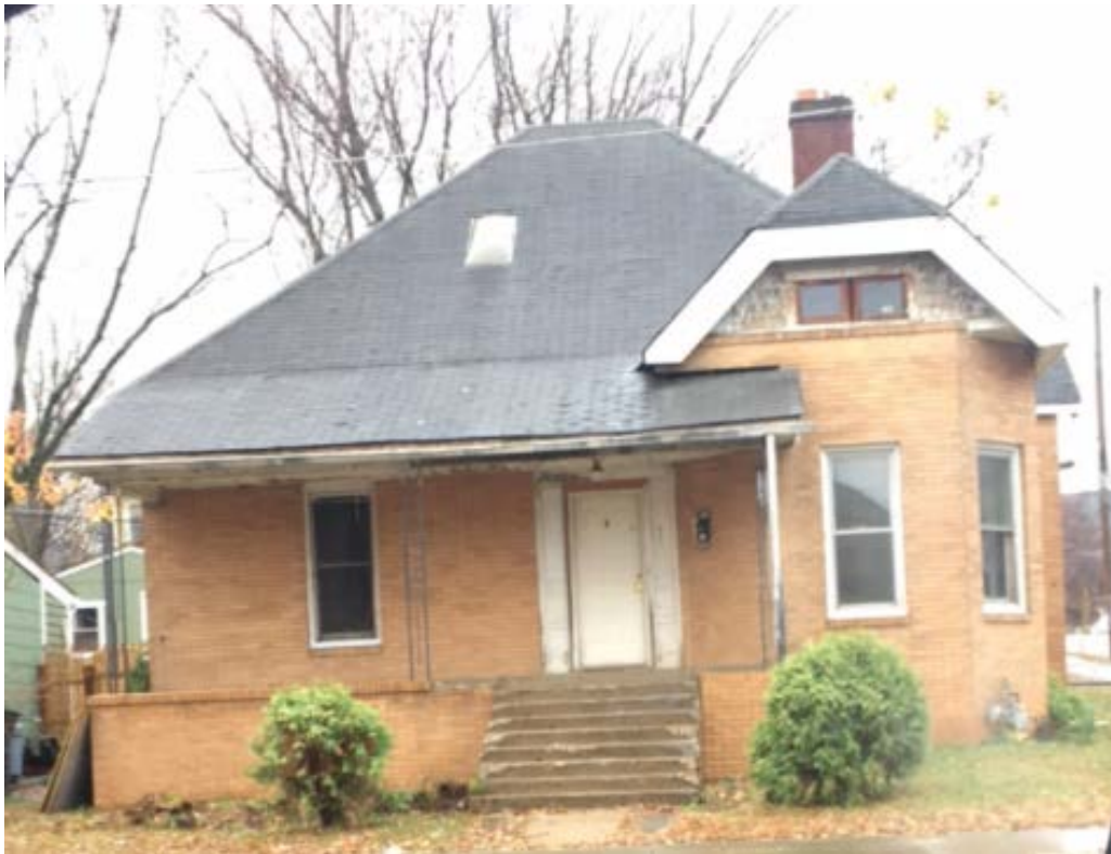
629 Luttrell Street - December 2016 - after work began
