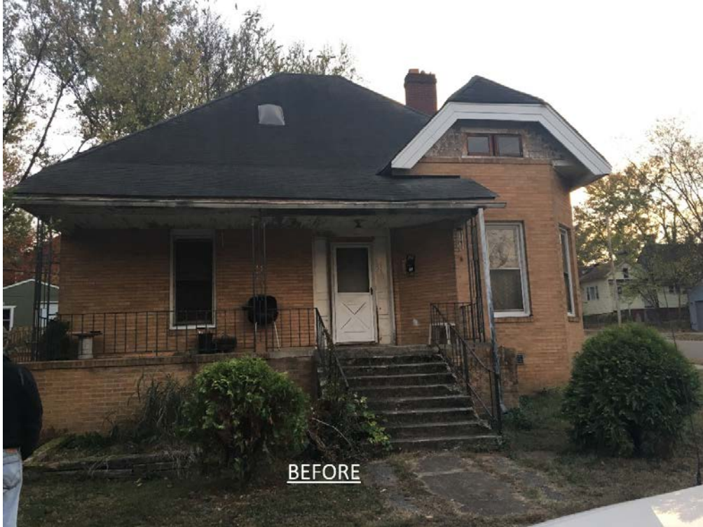
629 Luttrell Street- before work began
