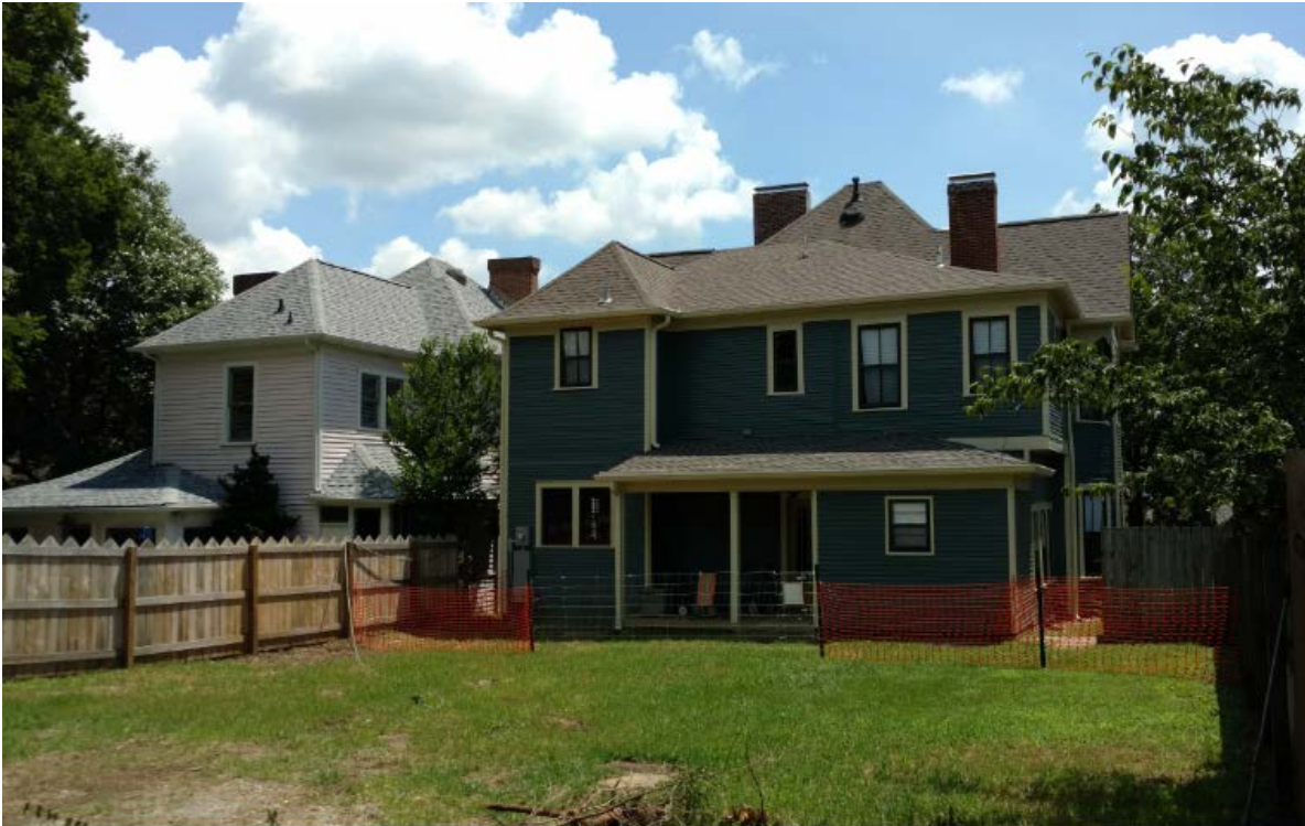
1019 Eleanor Street rear elevation showing location of garage to the right along alley
