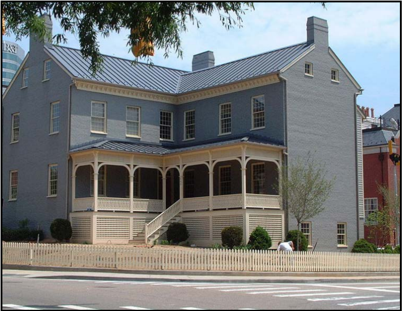
James Park House at 422 Cumberland Avenue constructed in 1812. This house exhibits a standing-seam type roof.
