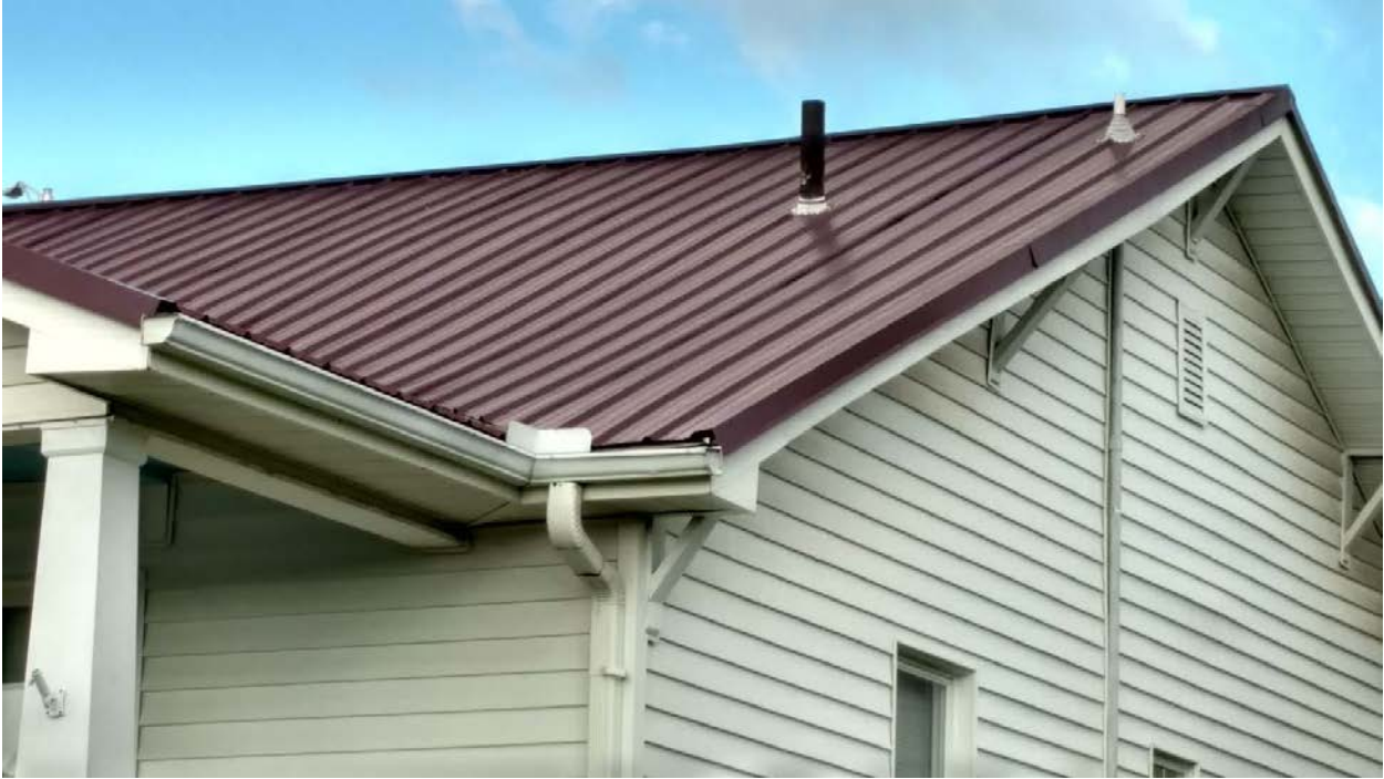
1317 N. 4th Ave. ribbed metal roofing (close-up)
