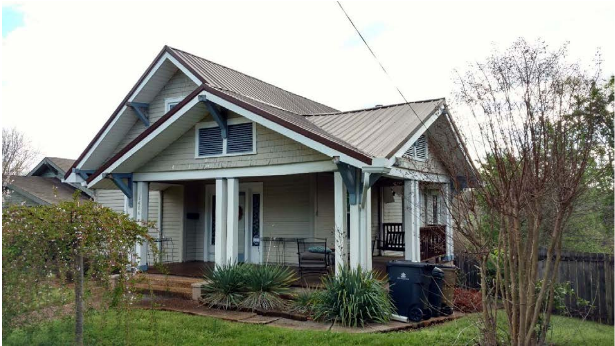
1406 N. 4th Ave. ribbed metal roofing (not in the H-1)
