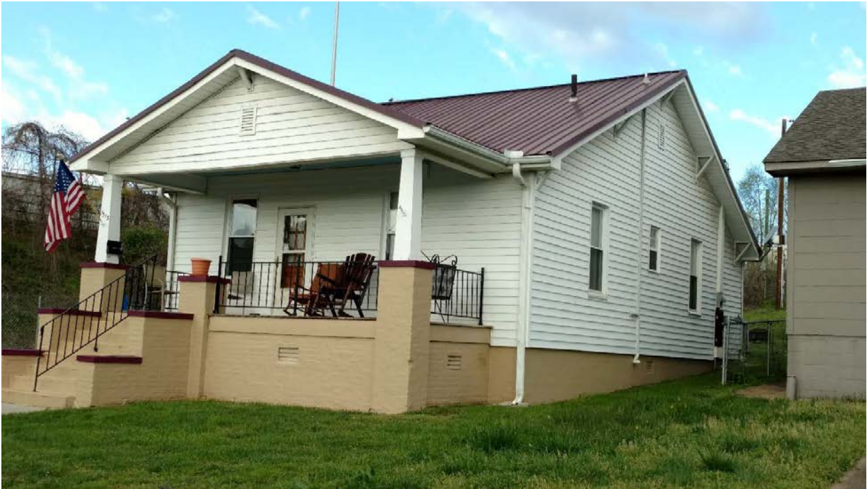
1317 N. 4th Ave. ribbed metal roofing (not in the H-1)
