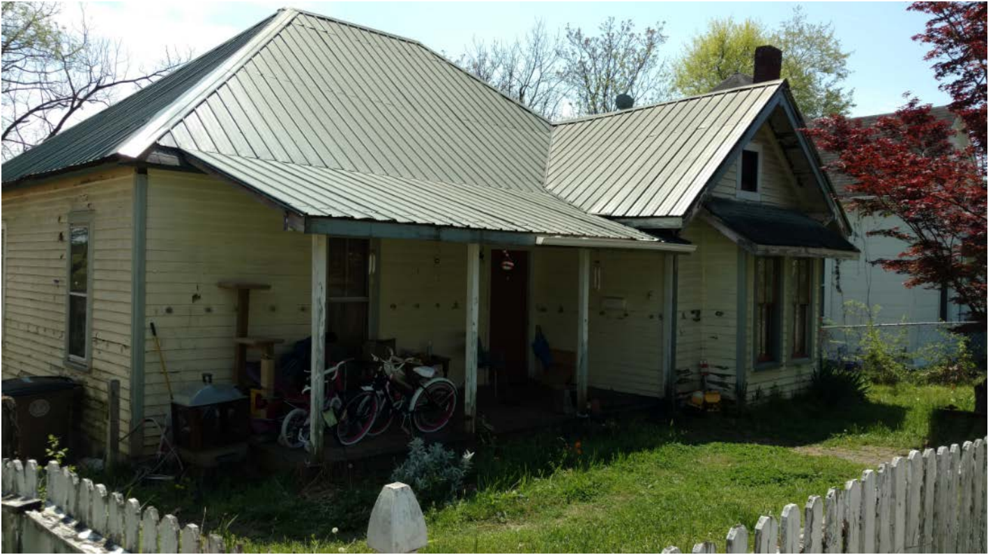
316 E. Scott Avenue in ONK with ribbed metal roofing (no COA)
