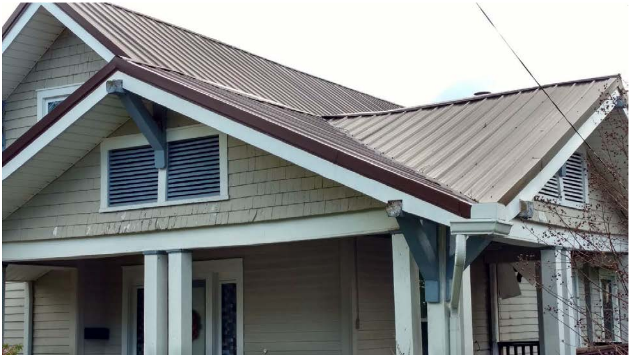
1406 N. 4th Ave. ribbed metal roofing (close-up)
