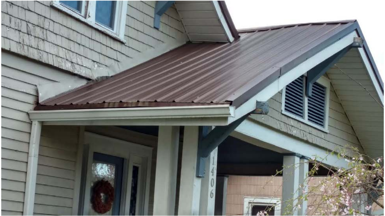
1406 N. 4th Ave. ribbed metal roofing (close-up showing edge profile)
