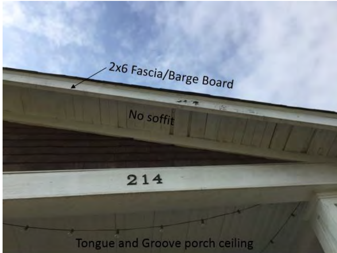
(Image 2) – Example of 2x6 fascia, no soffit, and tongue and groove porch ceiling on the front of the house (facing Northeast).
