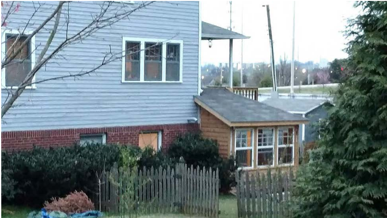
214 E. Glenwood - West facade showing addition
