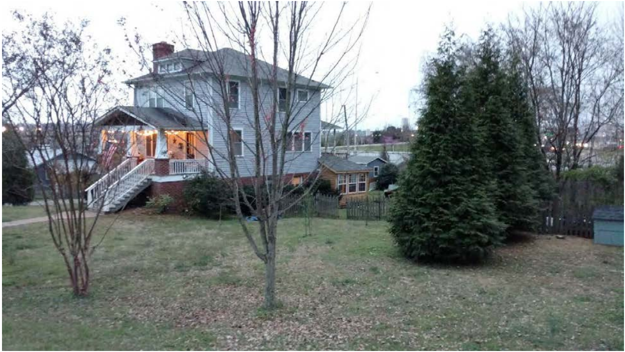
214 E. Glenwood - View from sidewalk
