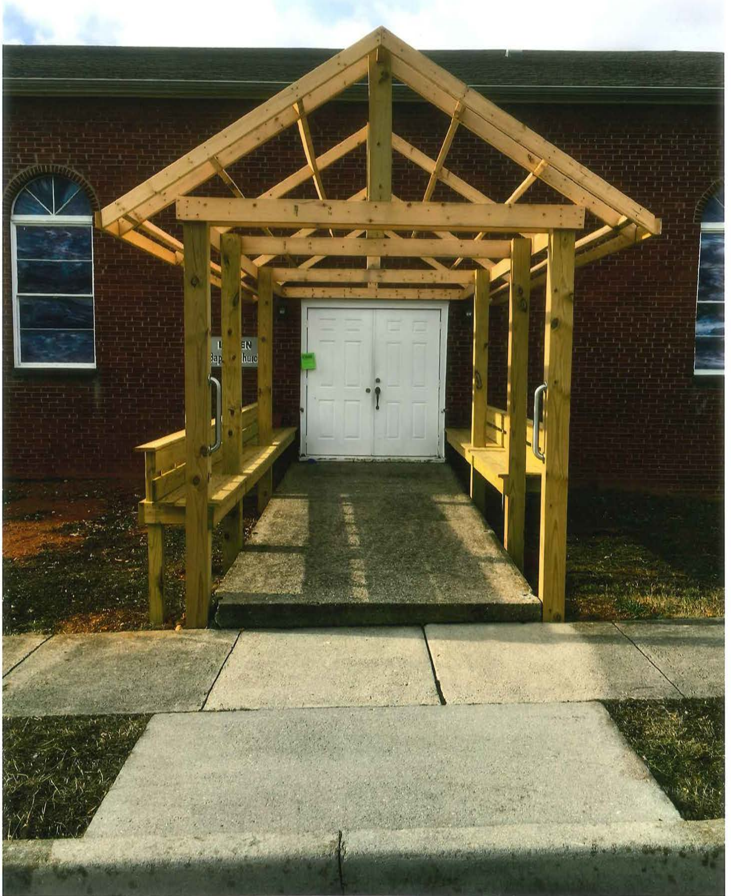
2341 Jefferson Ave - East elevation
