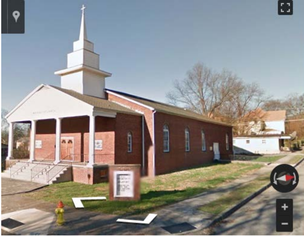
2342 Jefferson Avenue, corner of Spruce Avenue -Front and east facades
