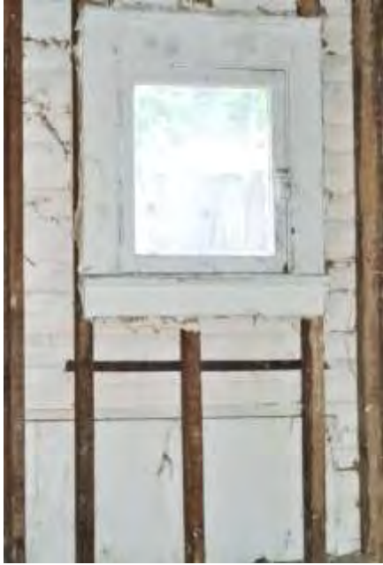
Highlight above left, original studs
