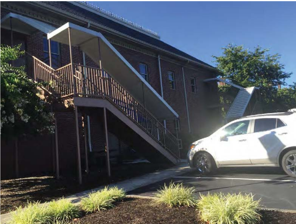
Existing Rear Entry (existing exterior stairs to be removed)
