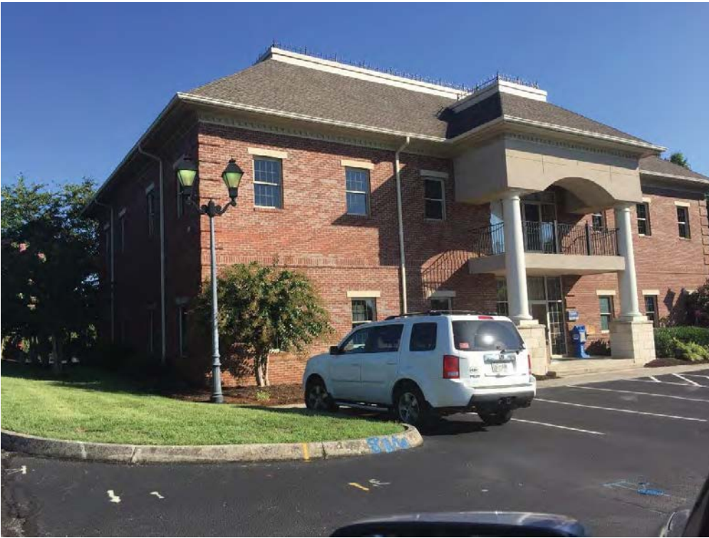
Existing Front Entry (to remain)
