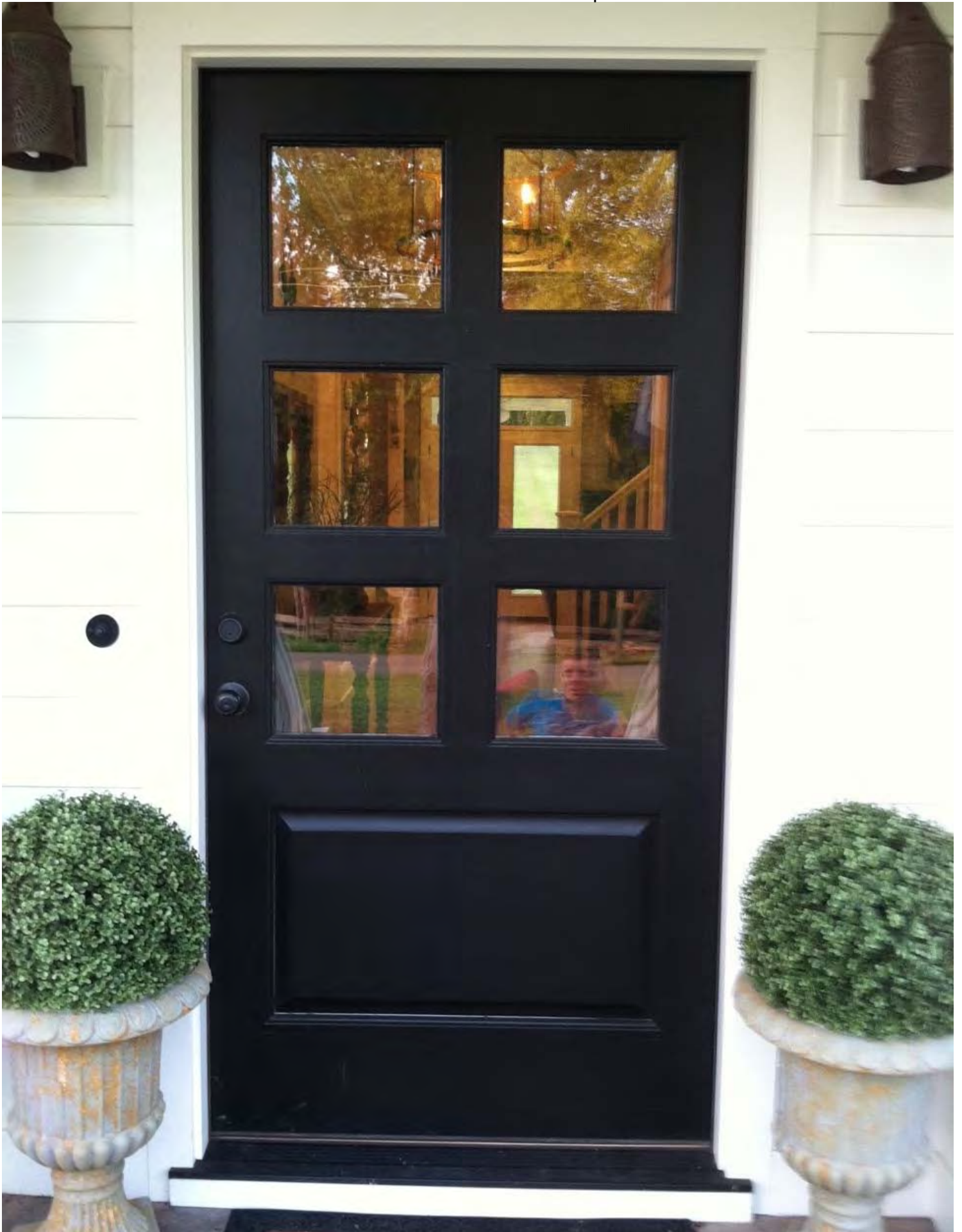
10721 Third Drive - Front door photo
