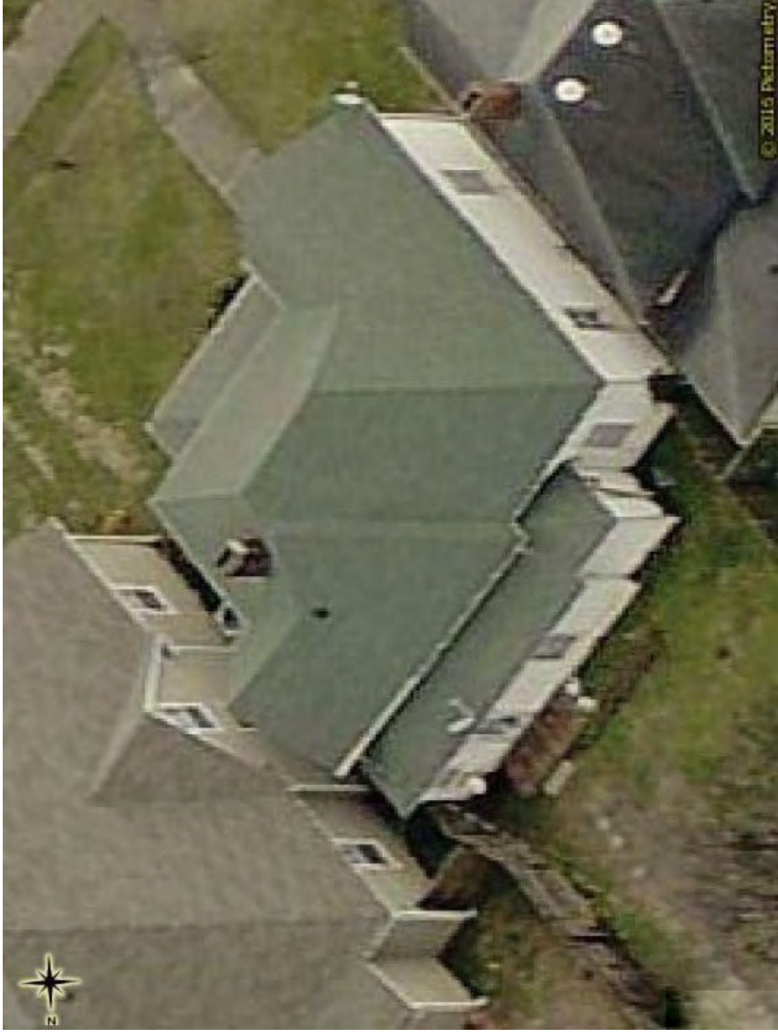
405 East Oklahoma NW side showing rear addition
