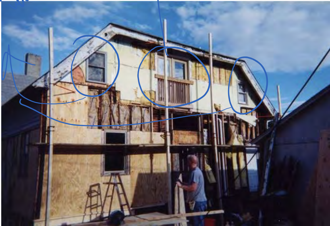
Fig. 2. This picture was taken after Fig. 1 probably in the 1990's, after the enclosed porch on the first floor had been removed. Two windows were put in on the second floor in the corners under the eaves of the roof, the four central windows were replaced with a French door; balcony would be put in soon after this photo.
