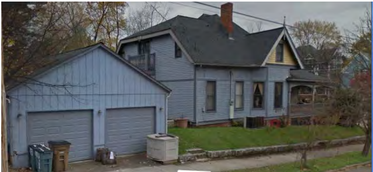
703 Luttrell – South facade
