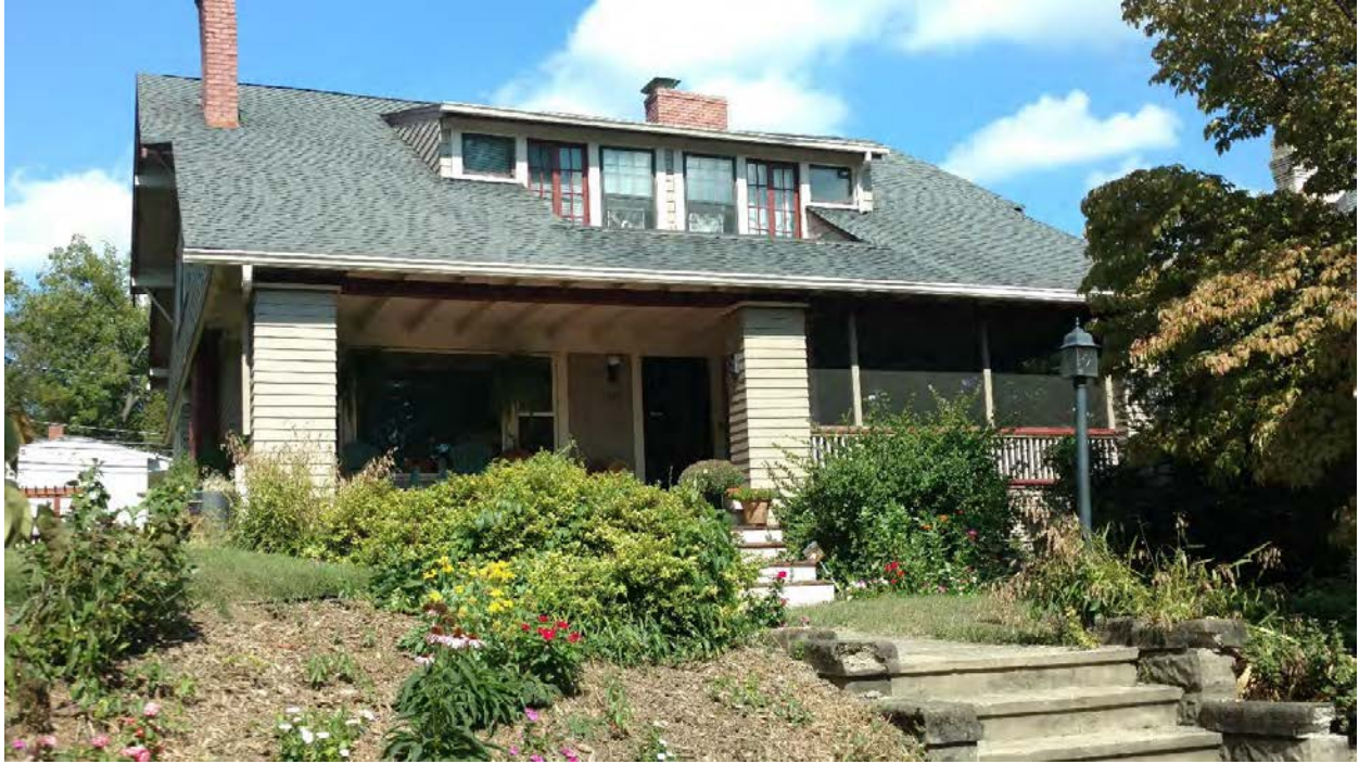
209 W. Glenwood Ave. – Front facade
