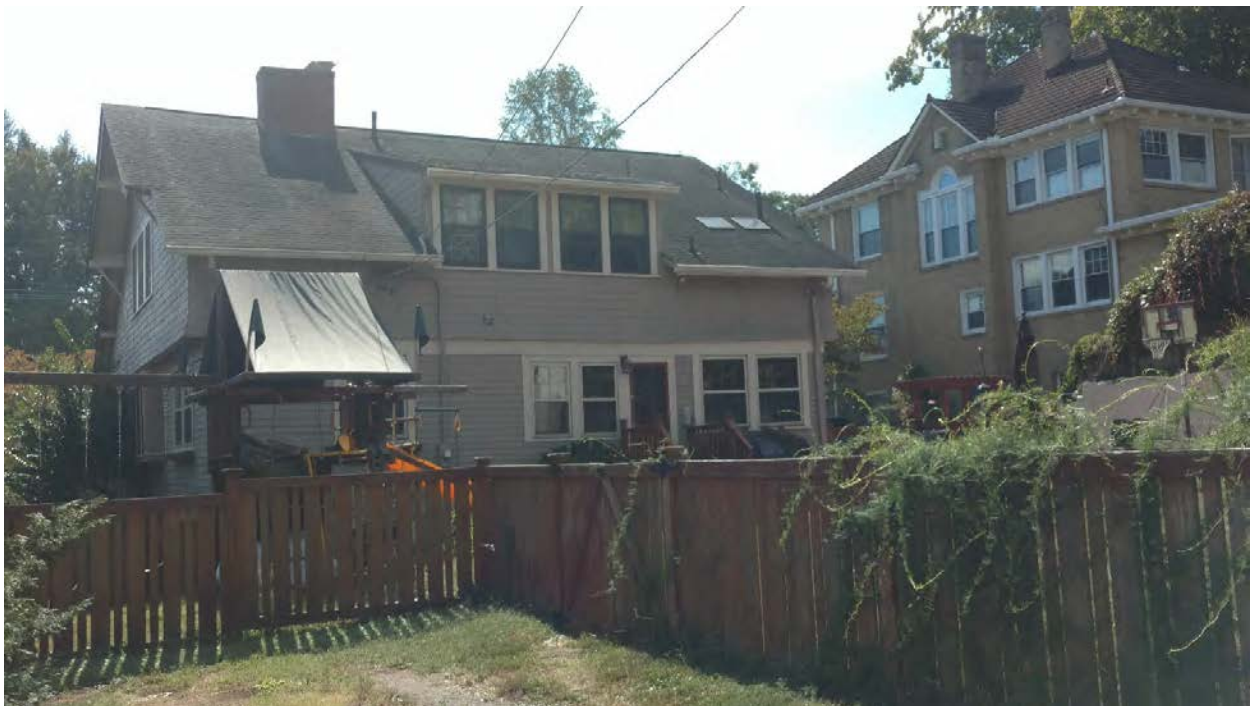
209 W. Glenwood Ave. – Rear façade looking southwest
