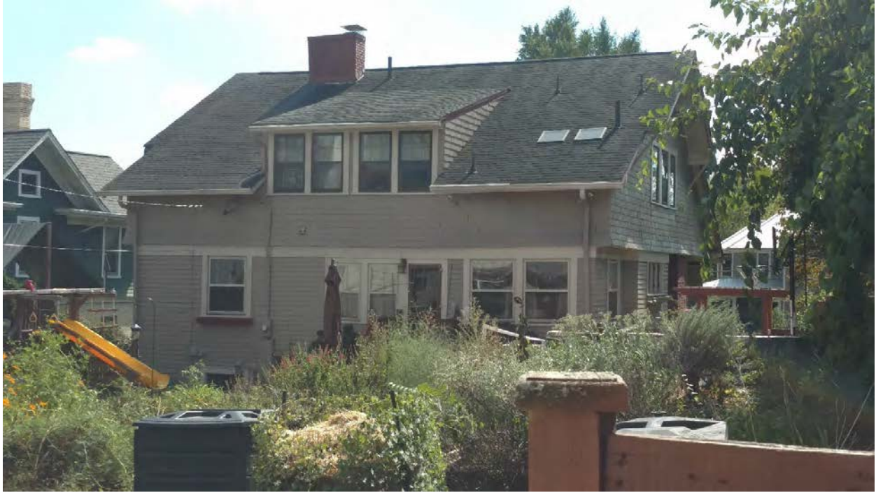
209 W. Glenwood Ave. – Rear façade looking southeast
