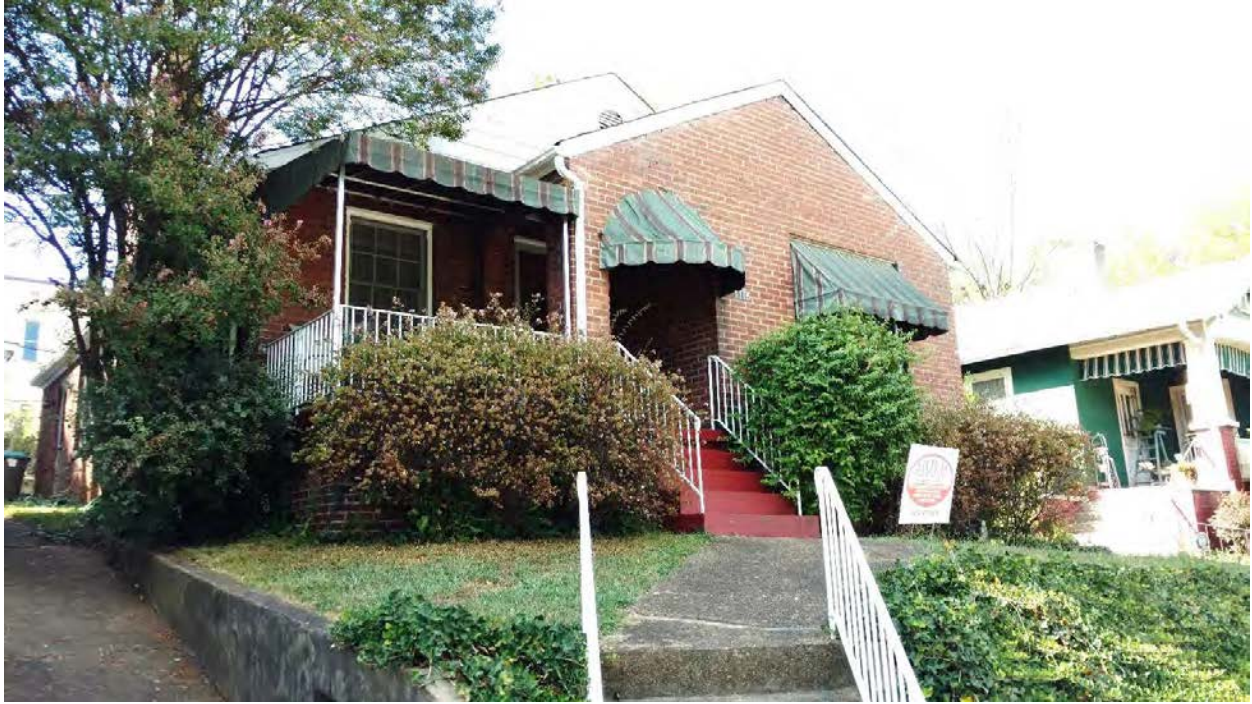
1115 Gratz Street - Front façade
