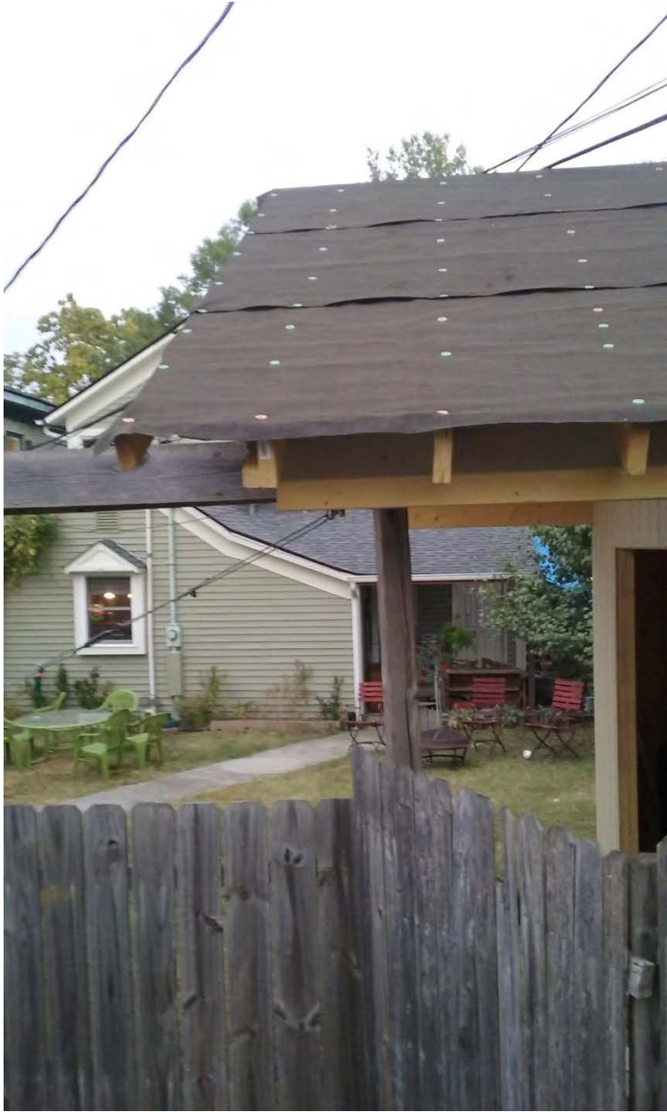
725 Deery - View of shed over fence in alley
