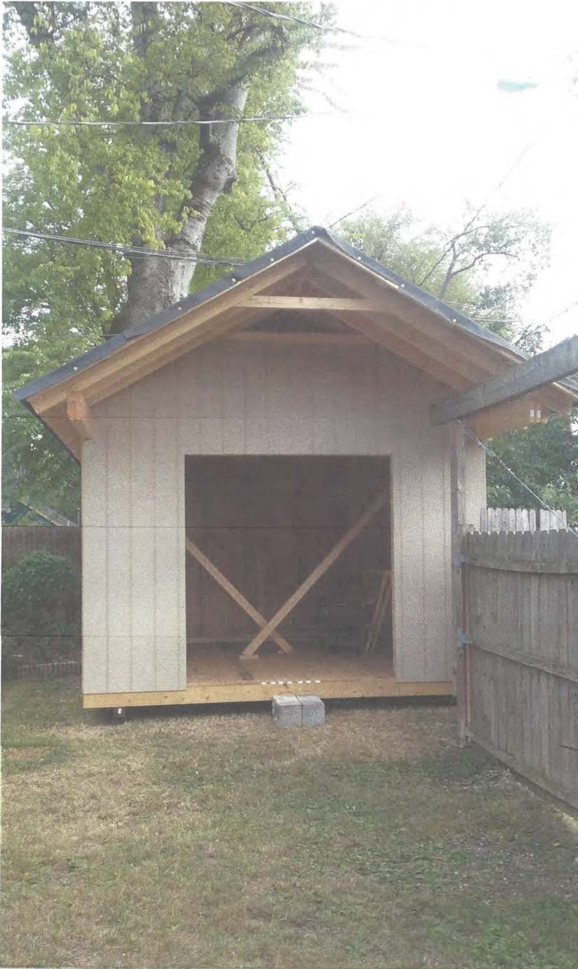
725 Deery - Front of outbuilding showing door opening
