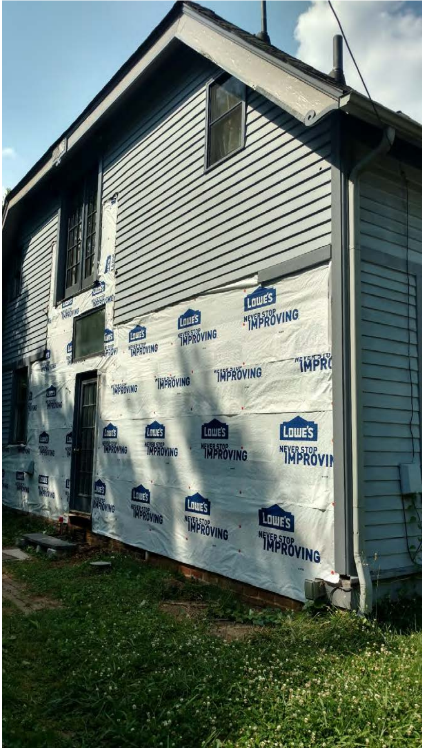
703 Luttrell – Current rear facade
