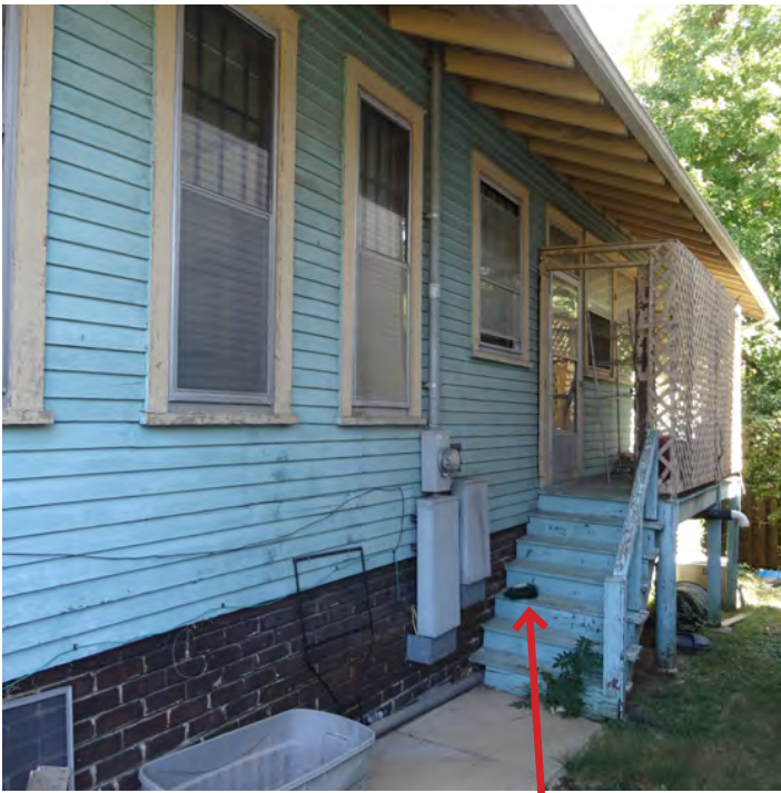
Painted wood replacement stair and handrail
