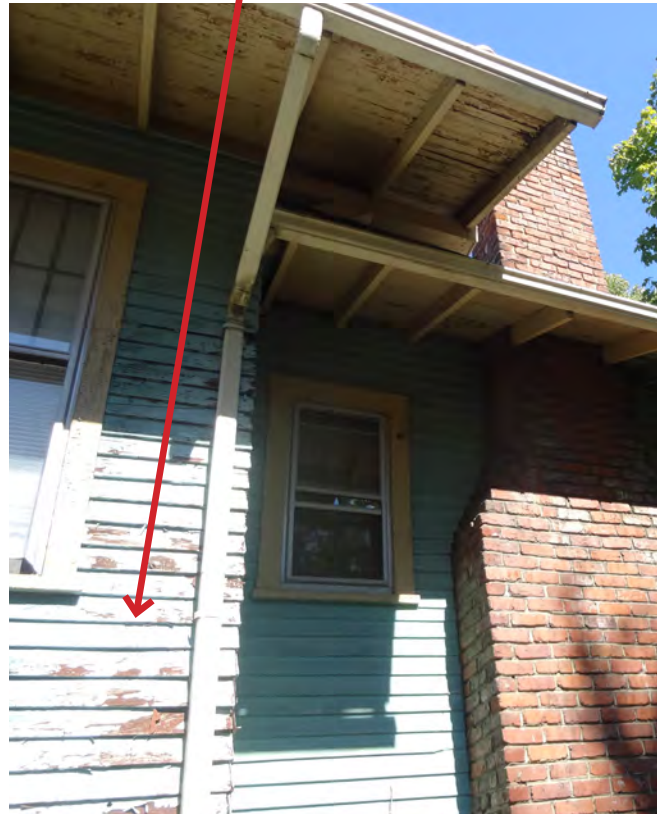
Some siding repair required on south side at back of house
