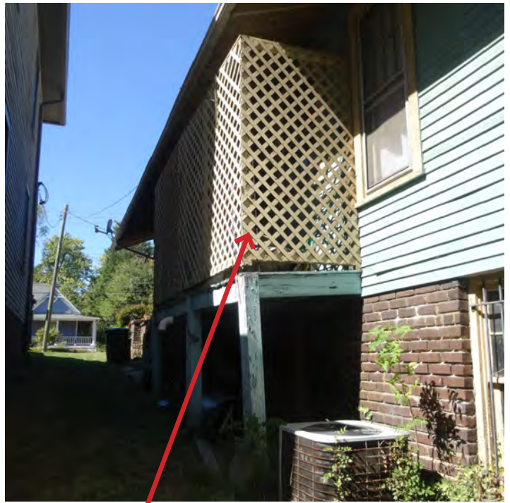
Replace deteriorated wood stair and lattice enclosure at kitchen door
