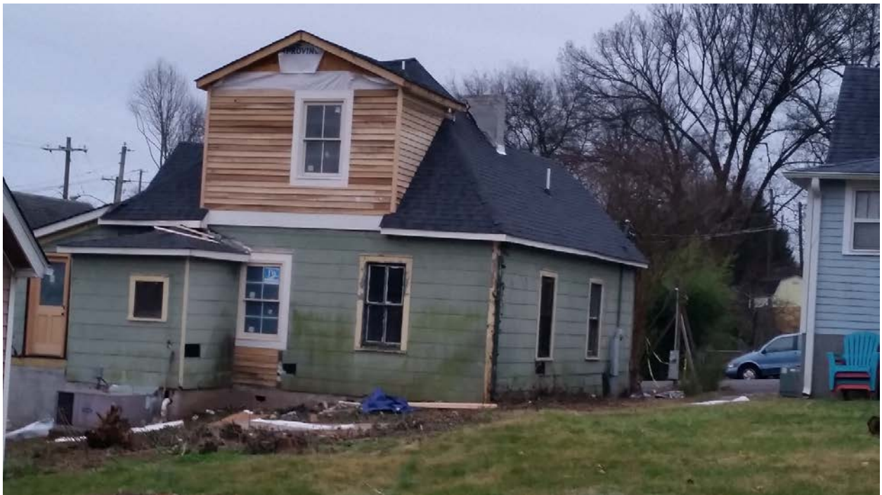
227 Leonard Place – Rear roof addition as seen from rear alley.
