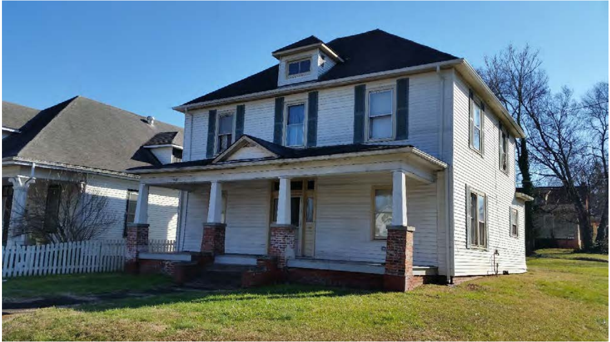
1400 Grainger Ave. – Front and west side from street corner
