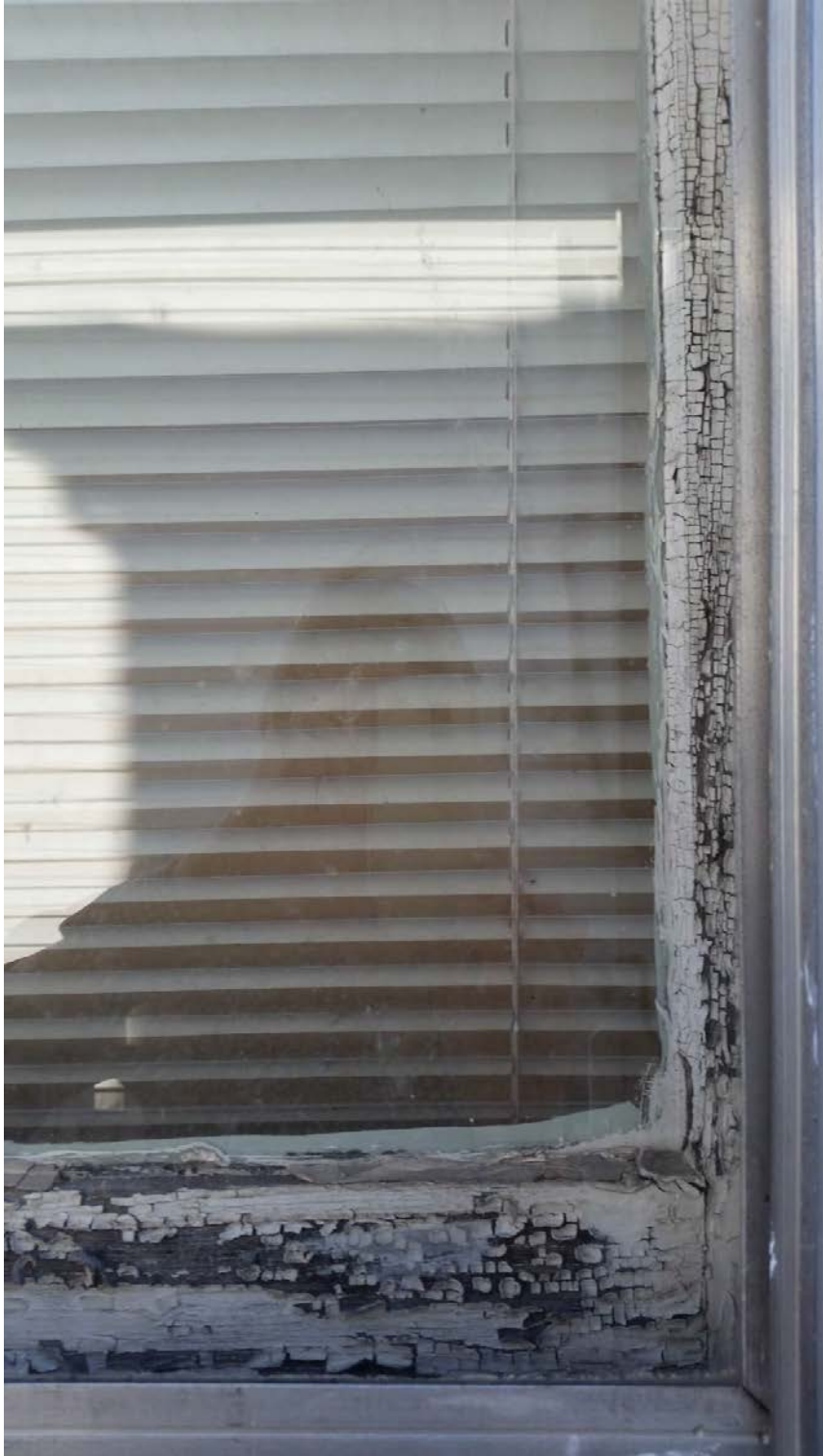
1400 Grainger Ave. – Original east side window to be replaced 2
