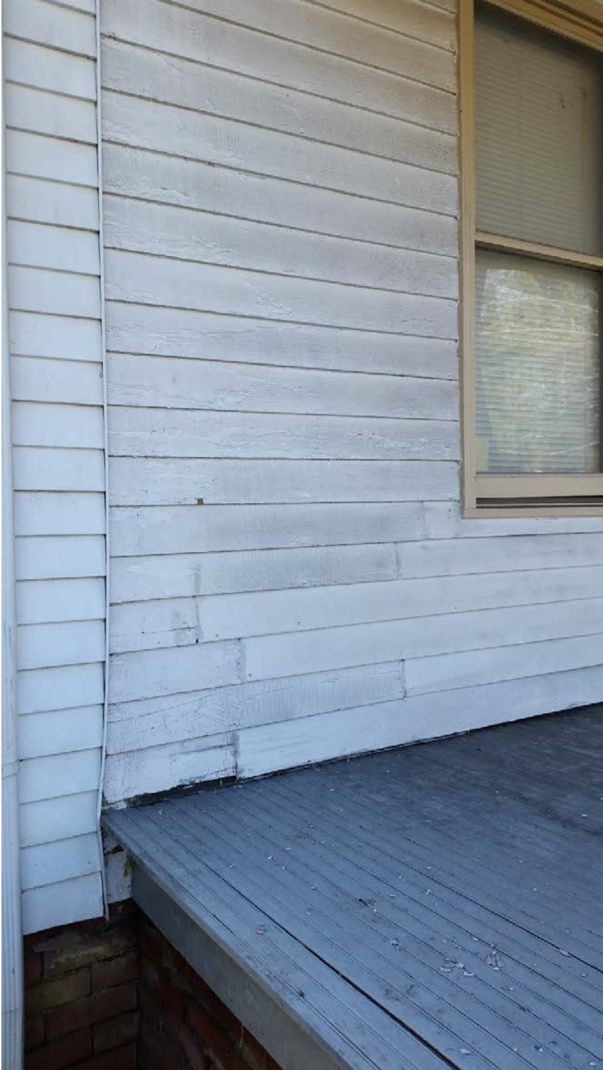
1400 Grainger Ave. – Aluminum siding to be removed
