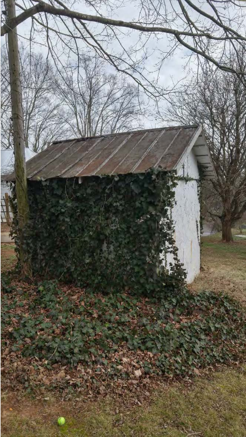
10913 Gilian Lane – Well house – north elevation
