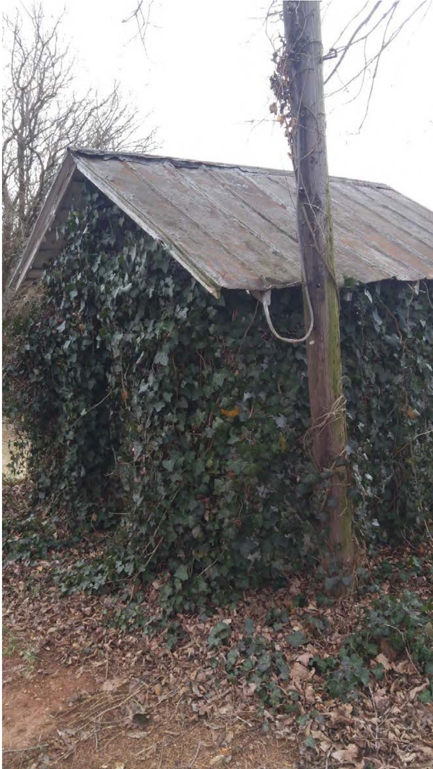
10913 Gilian Lane – Well house – east elevation
