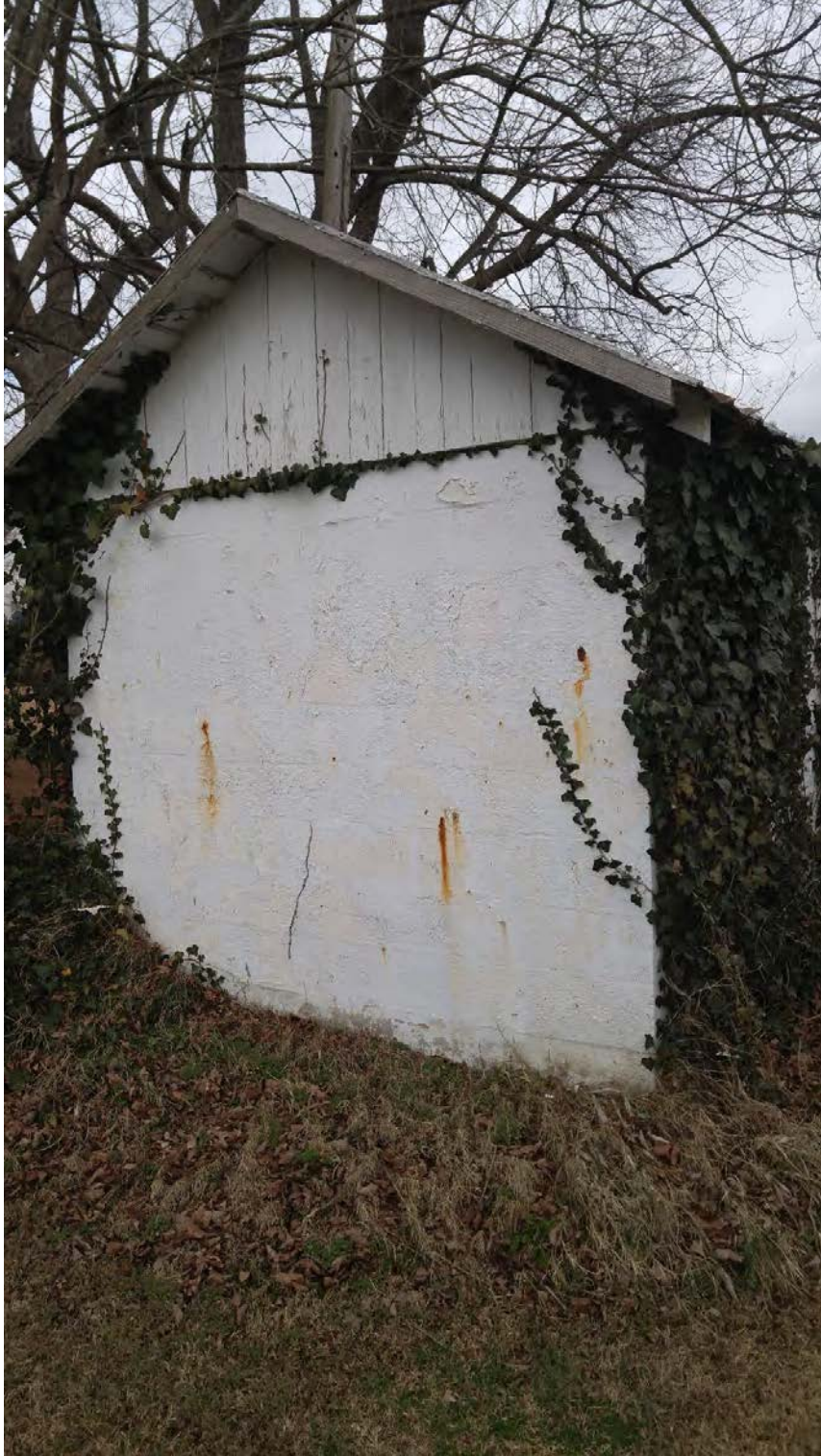
10913 Gilian Lane – Well house – west elevation
