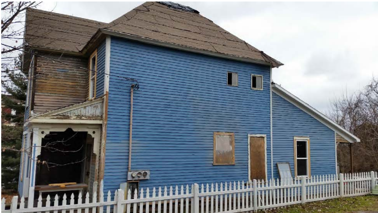
622 Deery St. – SE elevation from adjacent vacant lot
