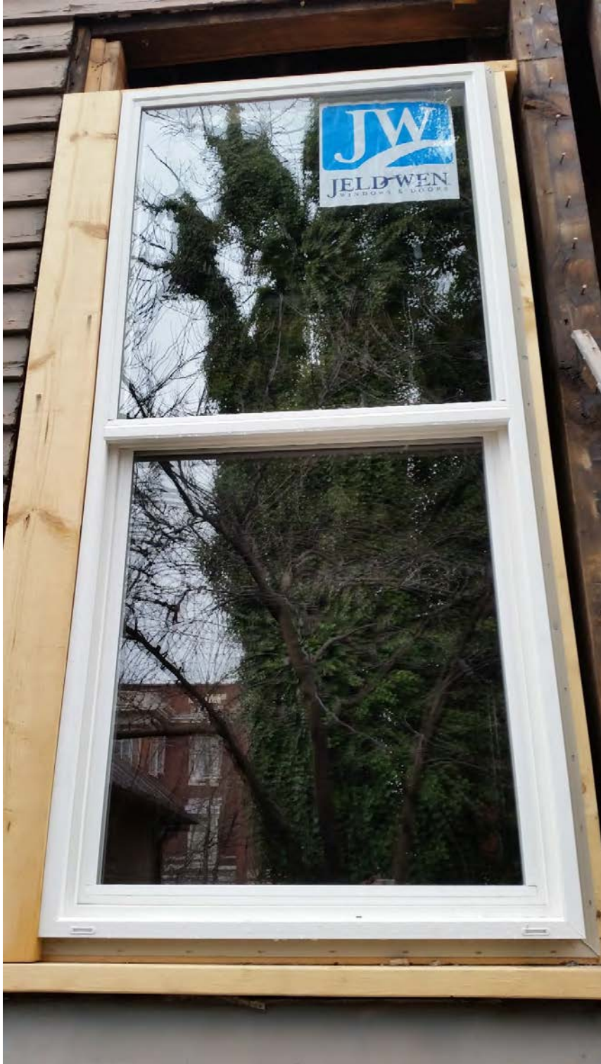
622 Deery St. – New vinyl window on 1 st level – NW side
