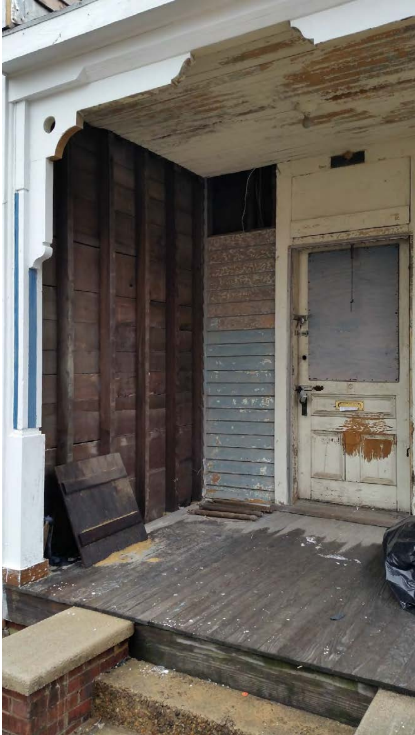
622 Deery St. – Front porch to be repaired in-kind
