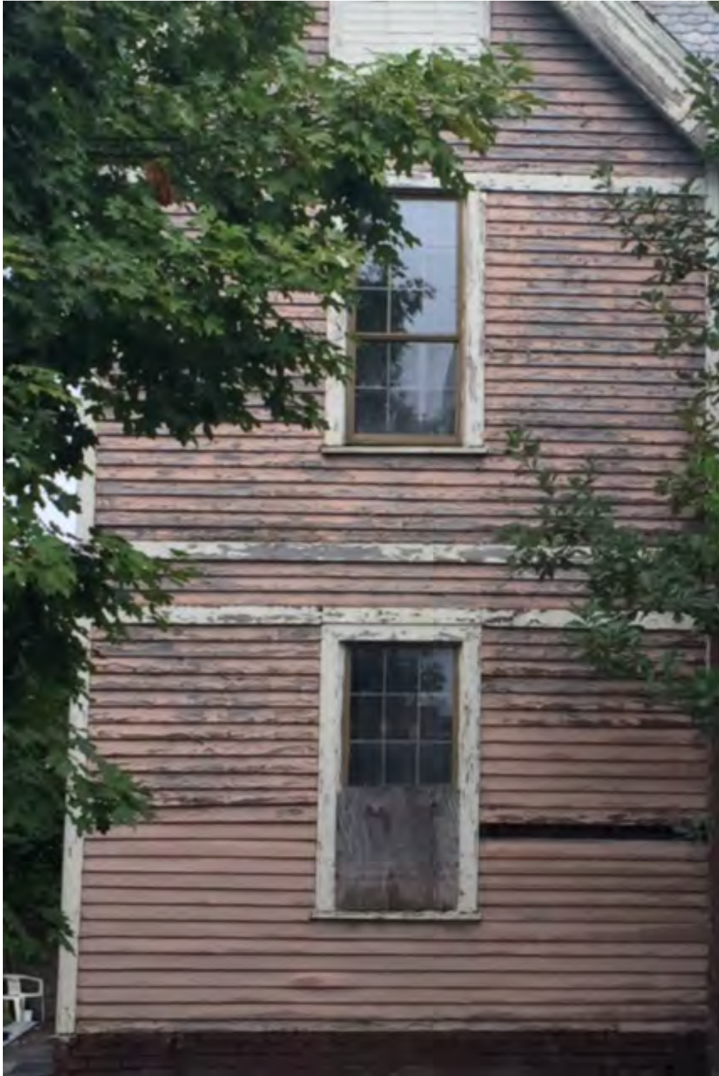
622 Deery St. – Front gable wing showing now removed widows
