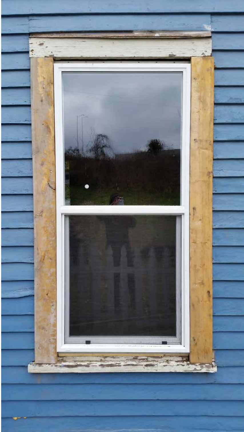
622 Deery St. – New vinyl window on 1 st level – SE elevation
