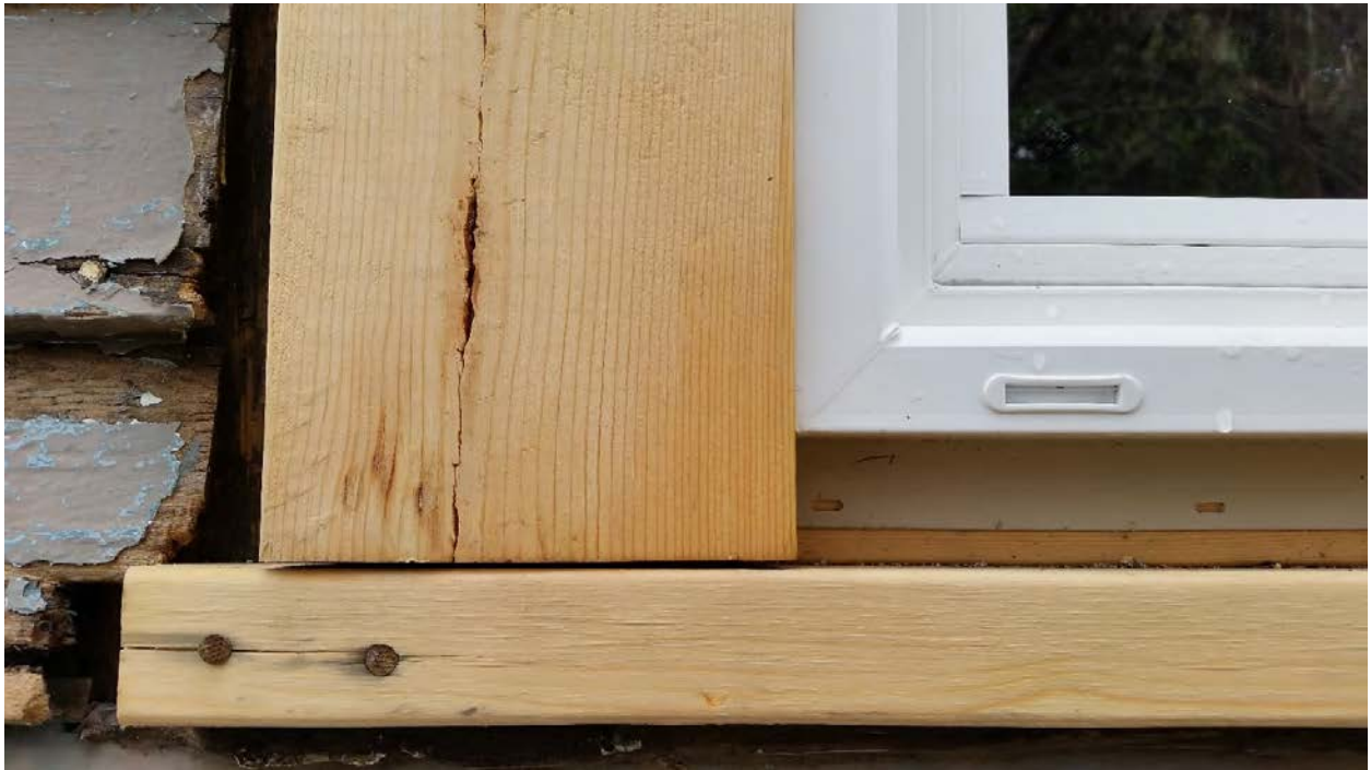
622 Deery St. – Close-up of new vinyl window on NW side
