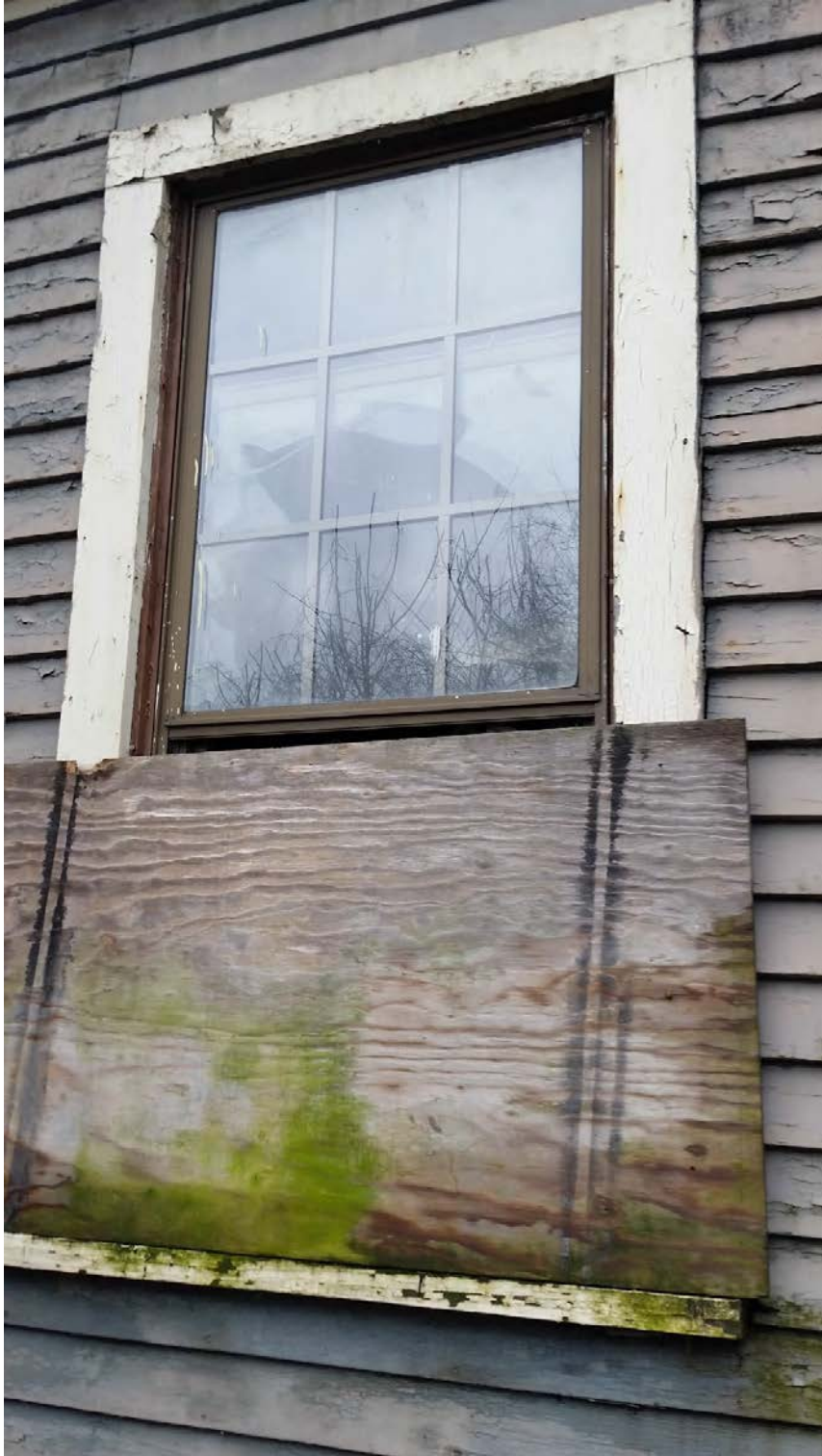
622 Deery St. – Metal window on SE side – now removed
