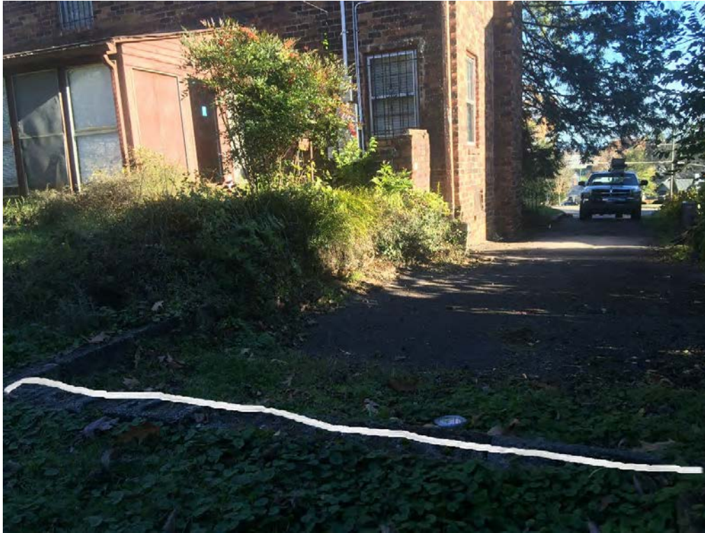
517 Oklahoma – Accessory structure location at end of driveway
