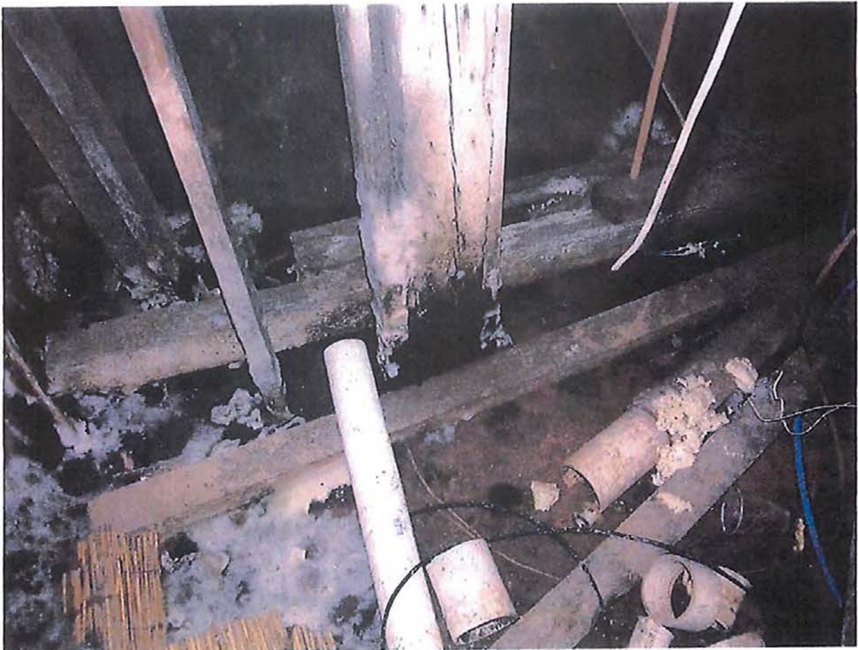
Typical post used to support the main level floor framing.
