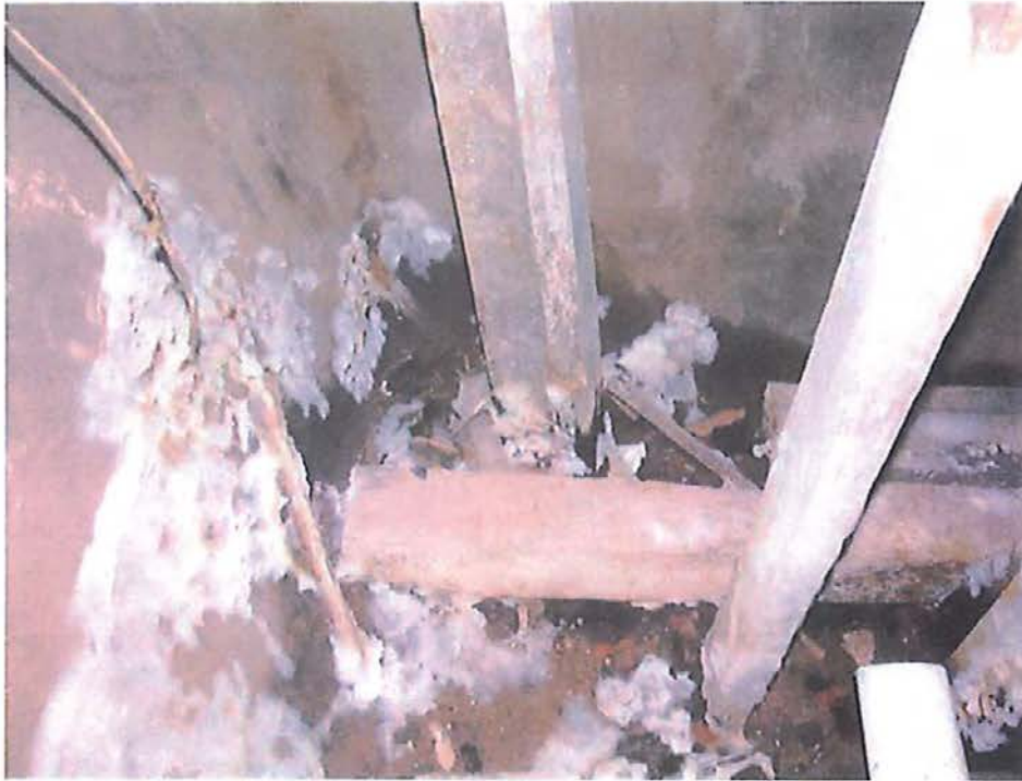
Posts and studs used to support the main level floor framing.
