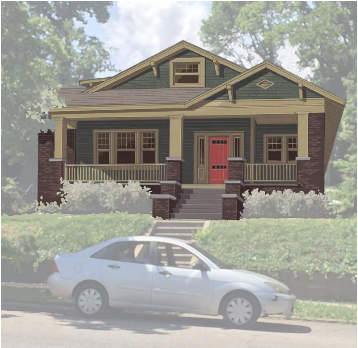
1819 White Avenue - Front view 2
