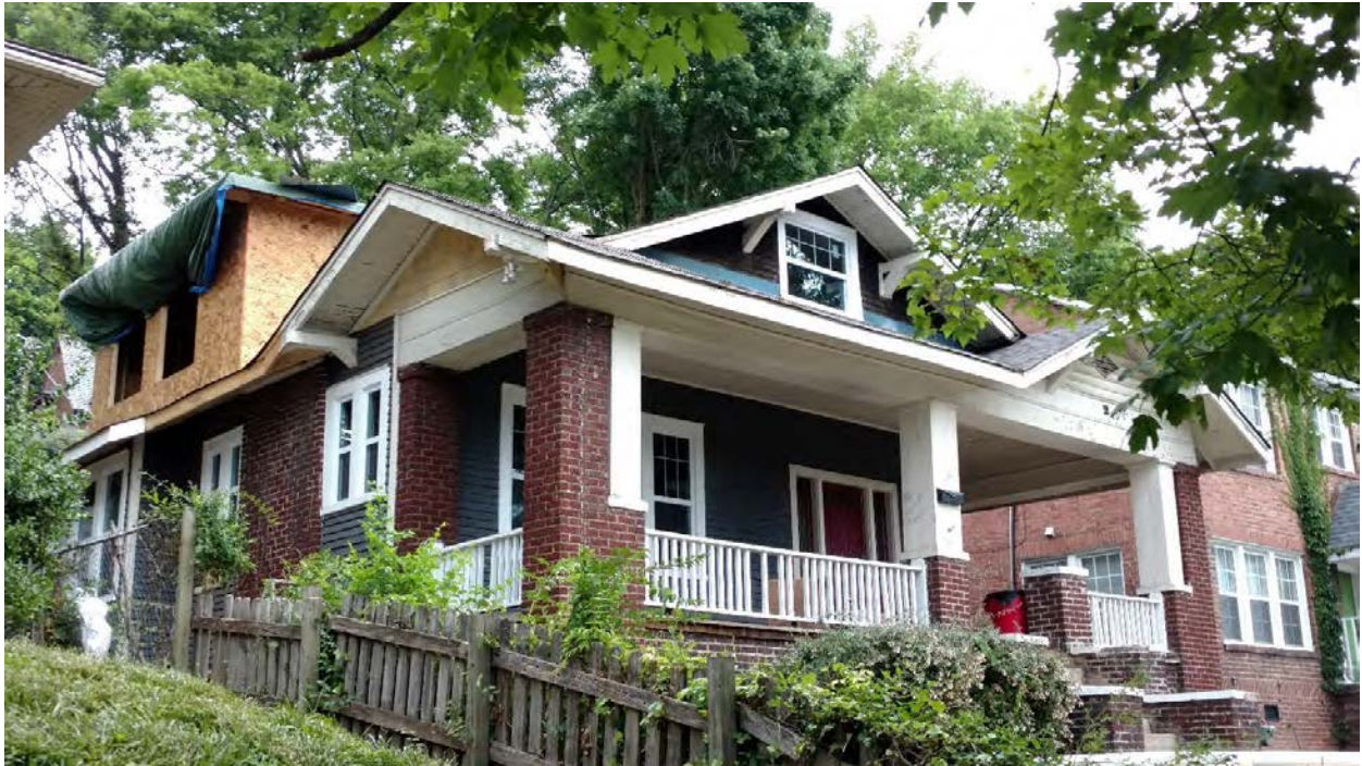
1819 White Avenue – View of partially constructed dormer from west
