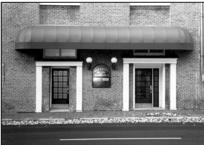
Side entrances with single continuous awning.
