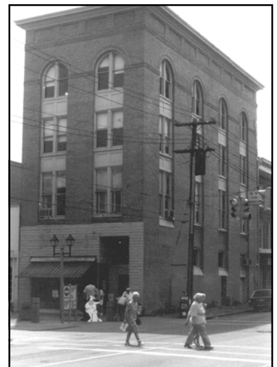
Building with permastone storefront prior to rehabilitation.
