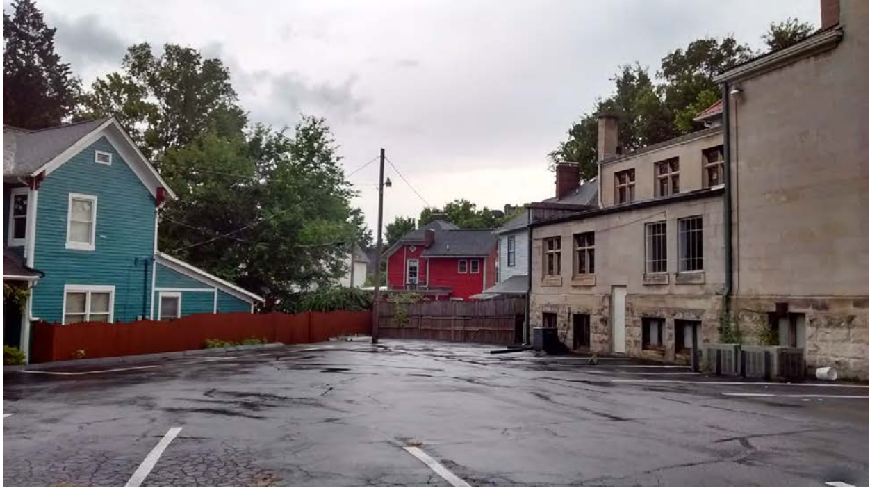
822 Deery Street - View of rear elevation (NE) of house from church parking lot
