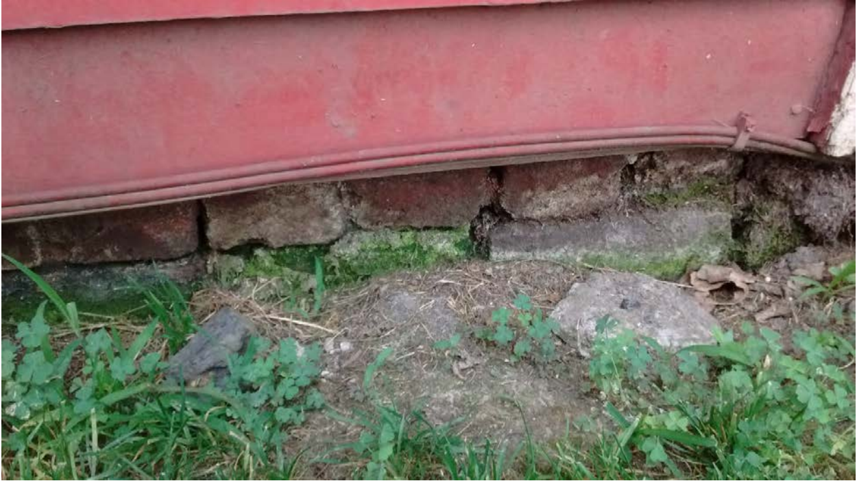
822 Deery Street - Brick foundation of house along rear
