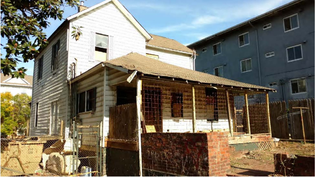
219 Twelfth St. – Northwest and rear façade
