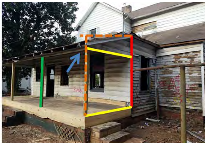
Figure 5: Flat view of the current roof Modification will alter the indicated roof by Raising the bottom portion of the roof from a current height Of 6'4" to 8' creating a new slope of 2/12
