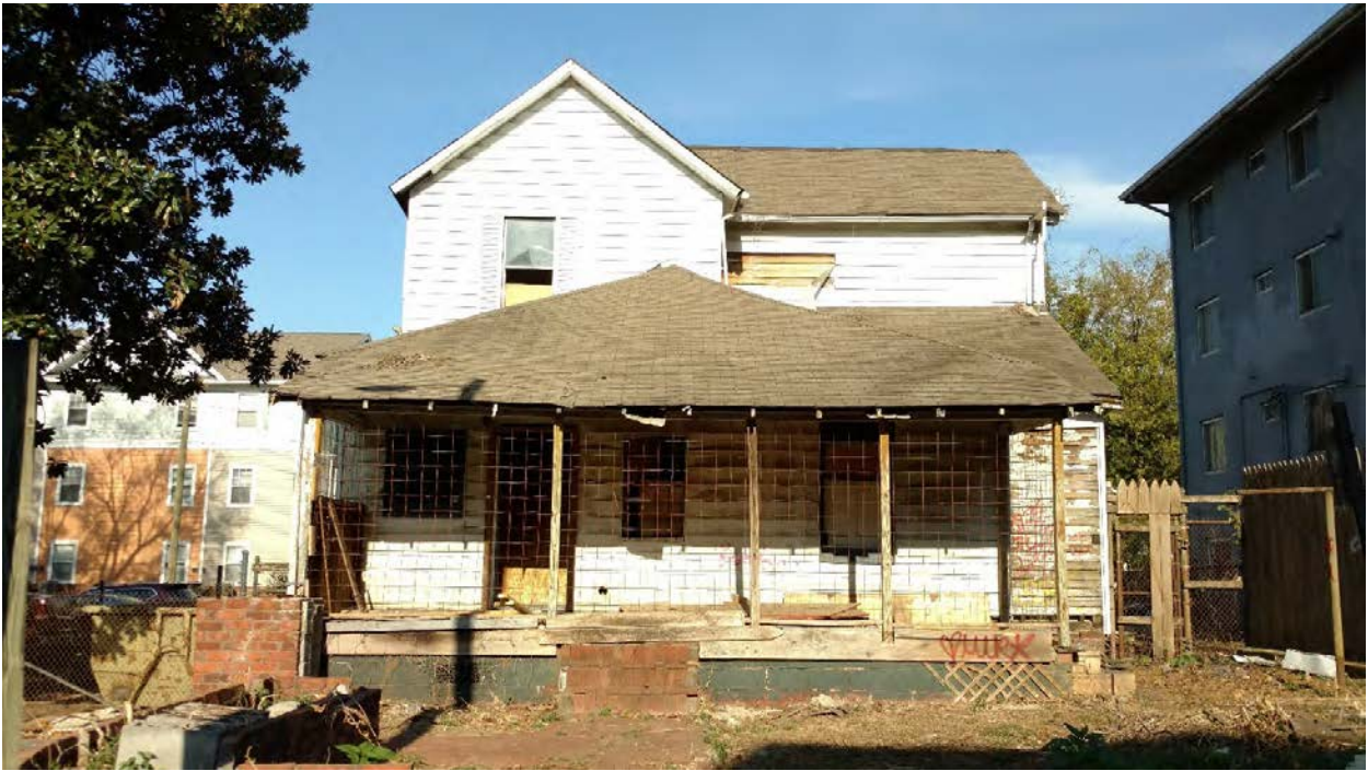
219 Twelfth St. – Rear facade
