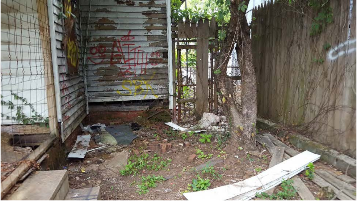
219 Twelfth St. – Rear southwest corner
