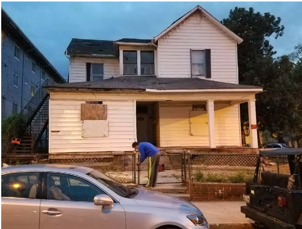
219 Twelfth St. - Front facade stabilization
