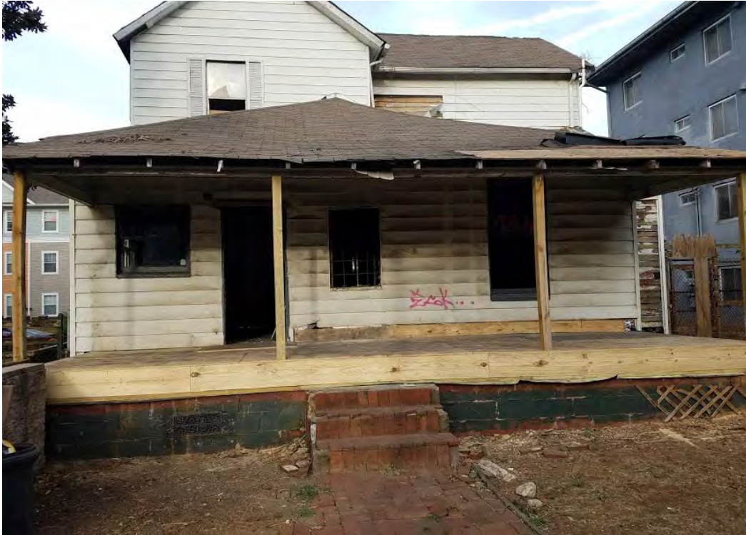
Figure 1. Current back of the House
