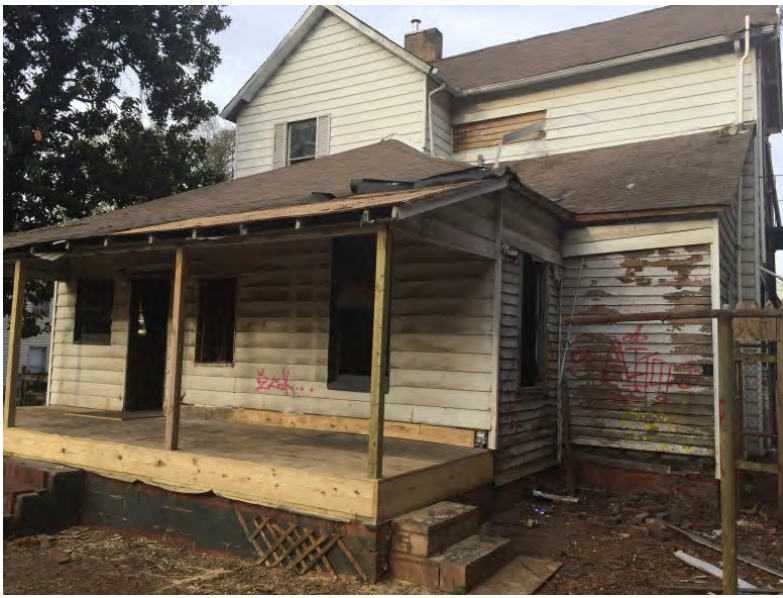
Figure 9. Existing view of southeast side
