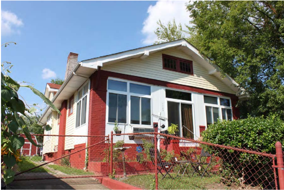
1709 Jefferson – Front and west facades as viewed from southwest on sidewalk
