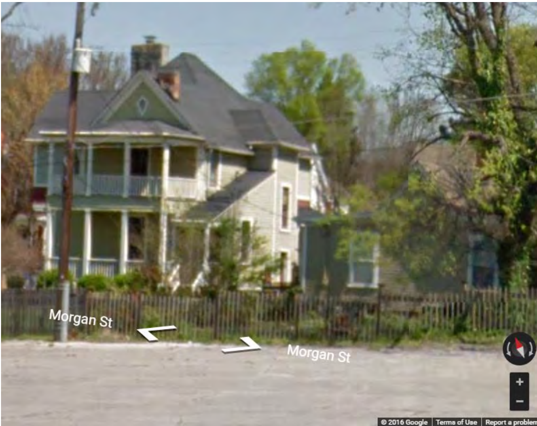
813 Deery Street rear façade as viewed from parking lot along Morgan Street - looking northwest
