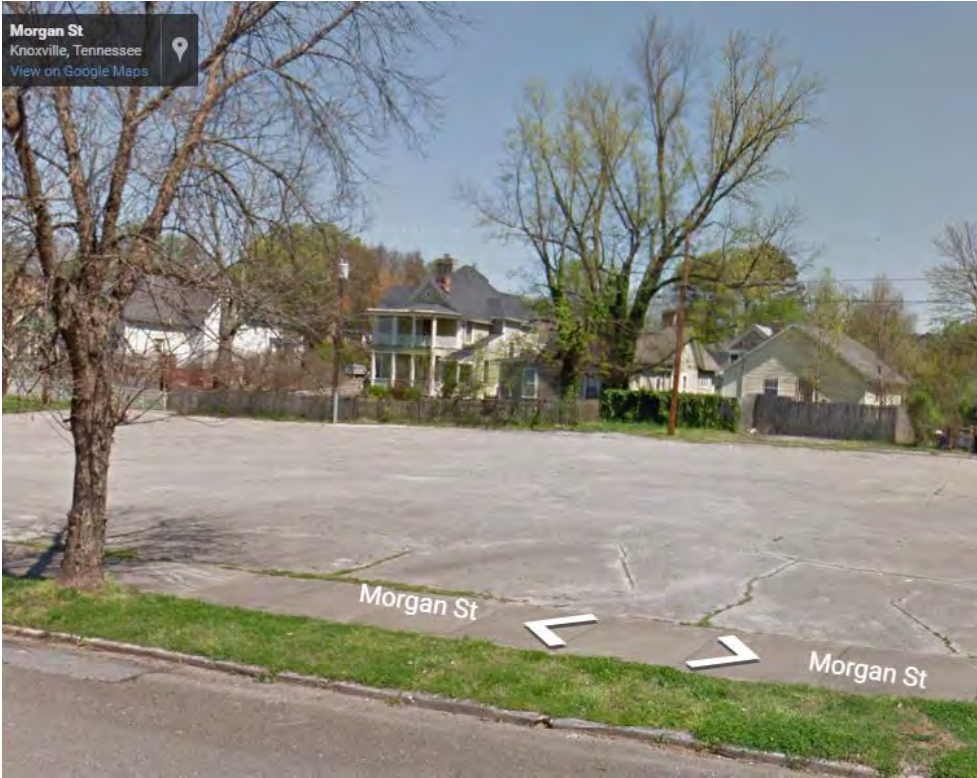
813 Deery Street rear façade as viewed from Morgan Street (~150 away)
