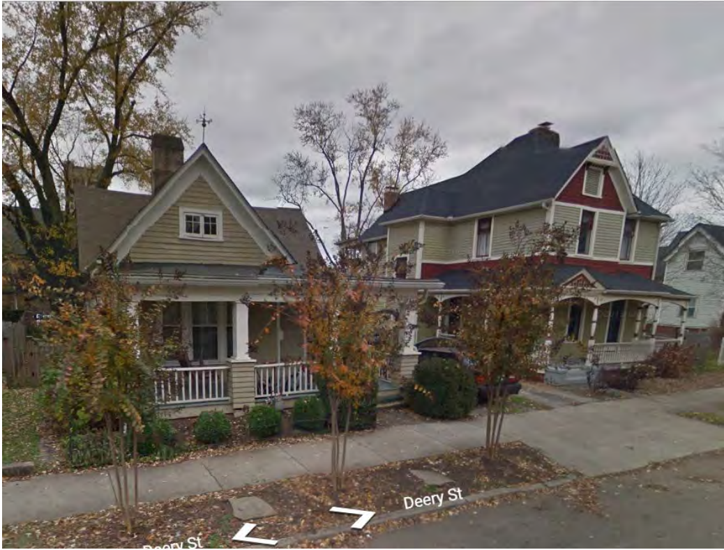
813 Deery Street showing the streetscape when approaching from the southeast
