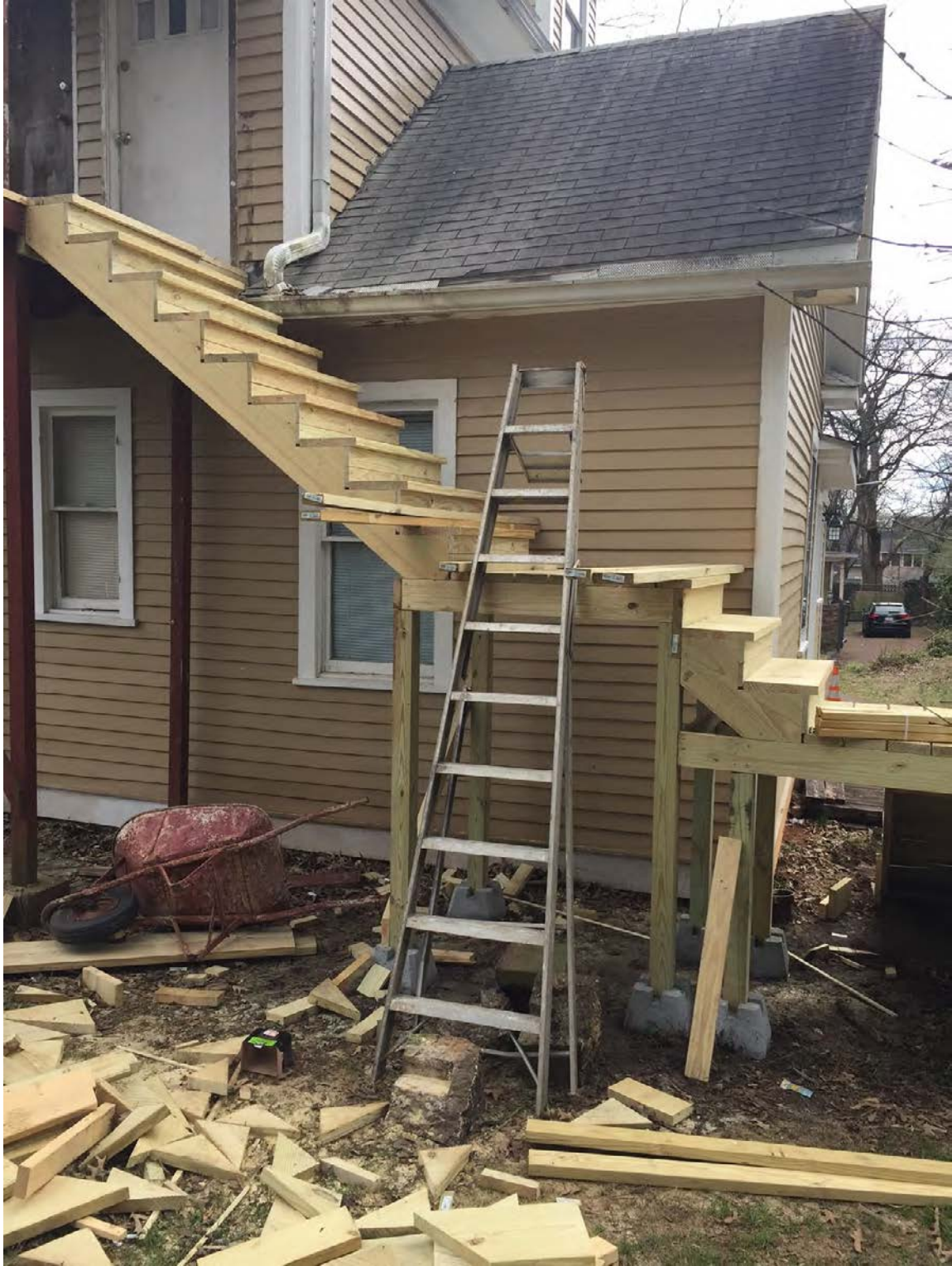
1335 Armstrong – New steps leading up to existing landing and door
