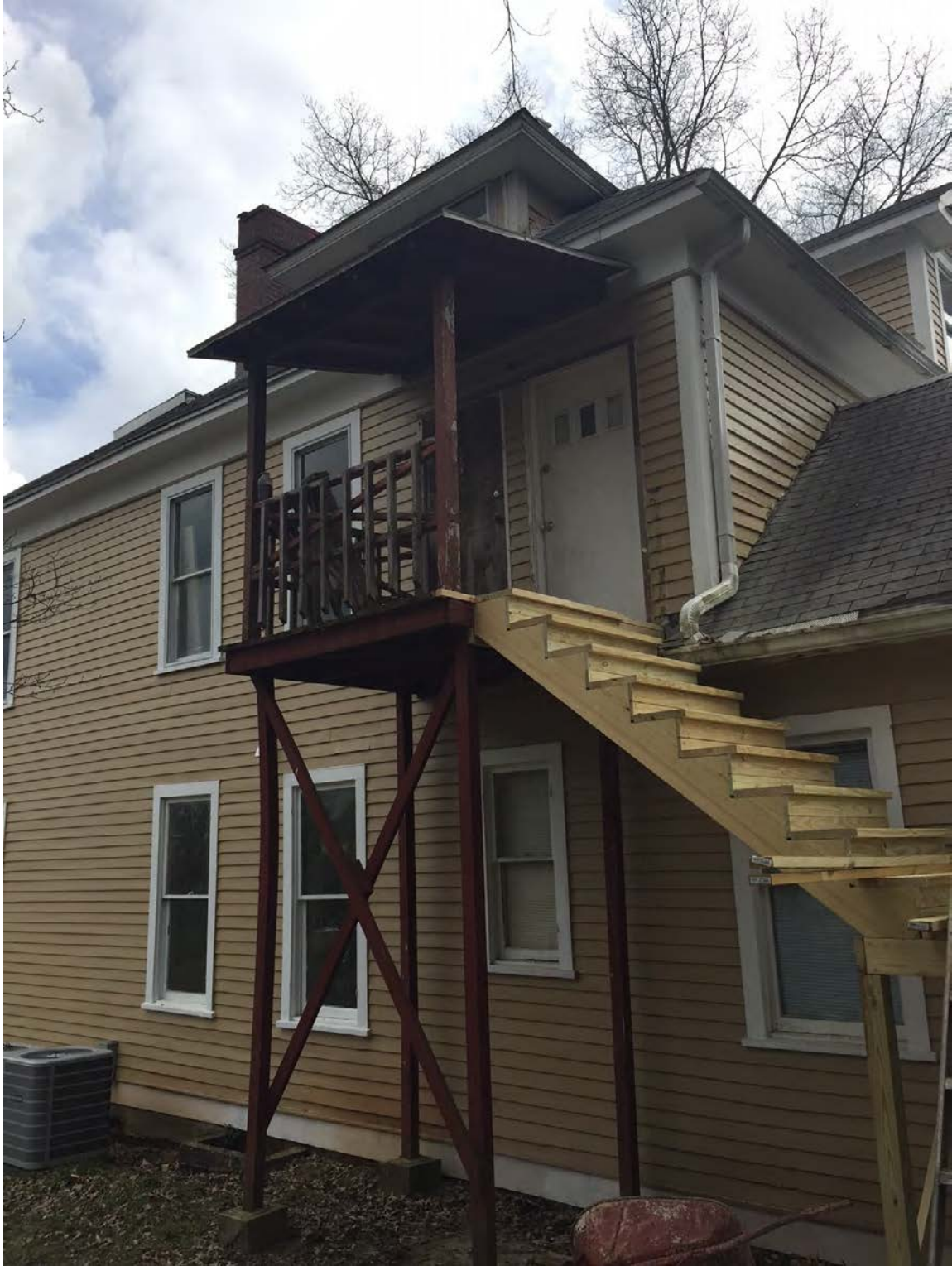
1335 Armstrong – New steps leading up to existing landing and door (2)
