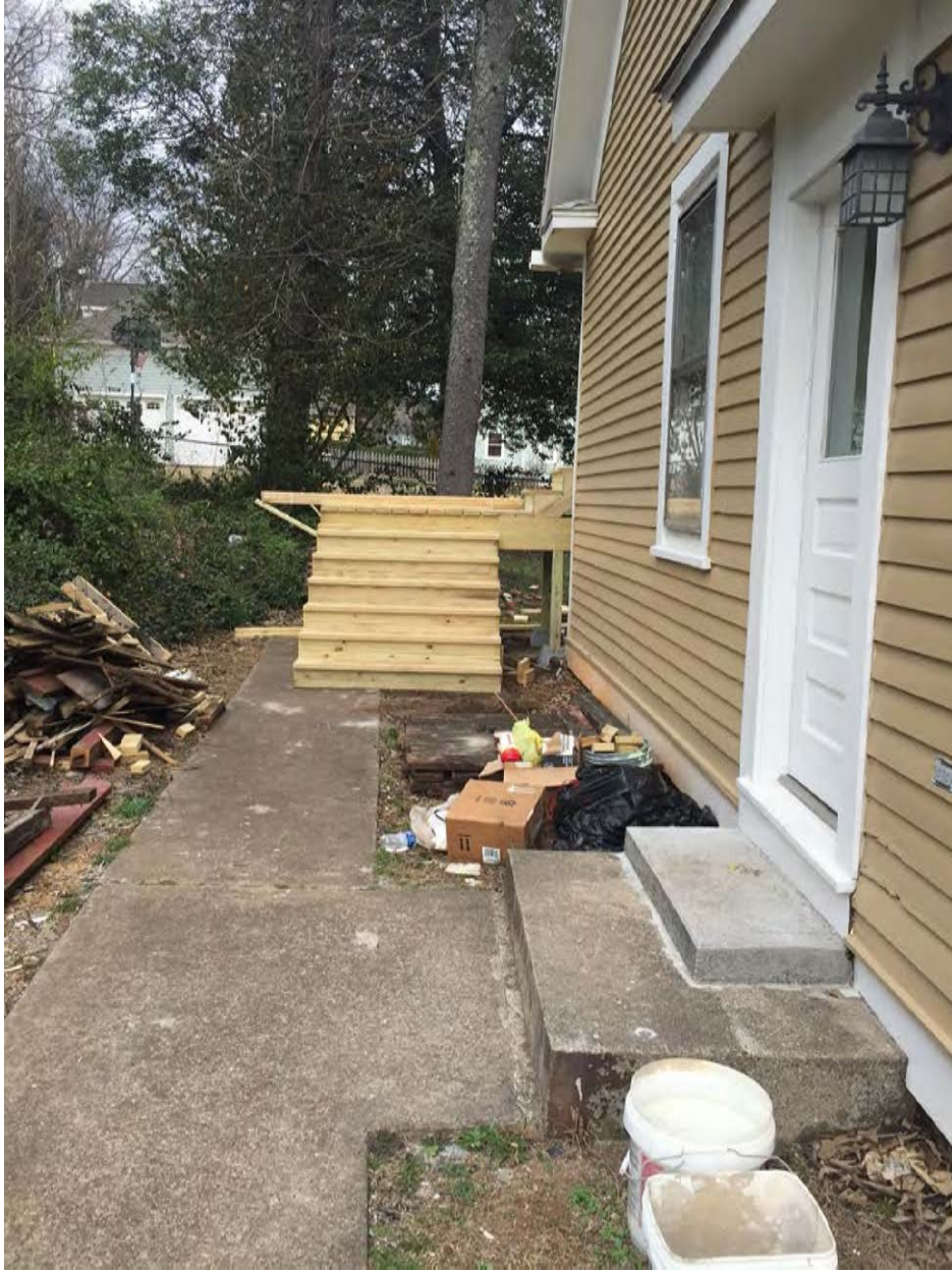
1335 Armstrong – View of steps from rear
